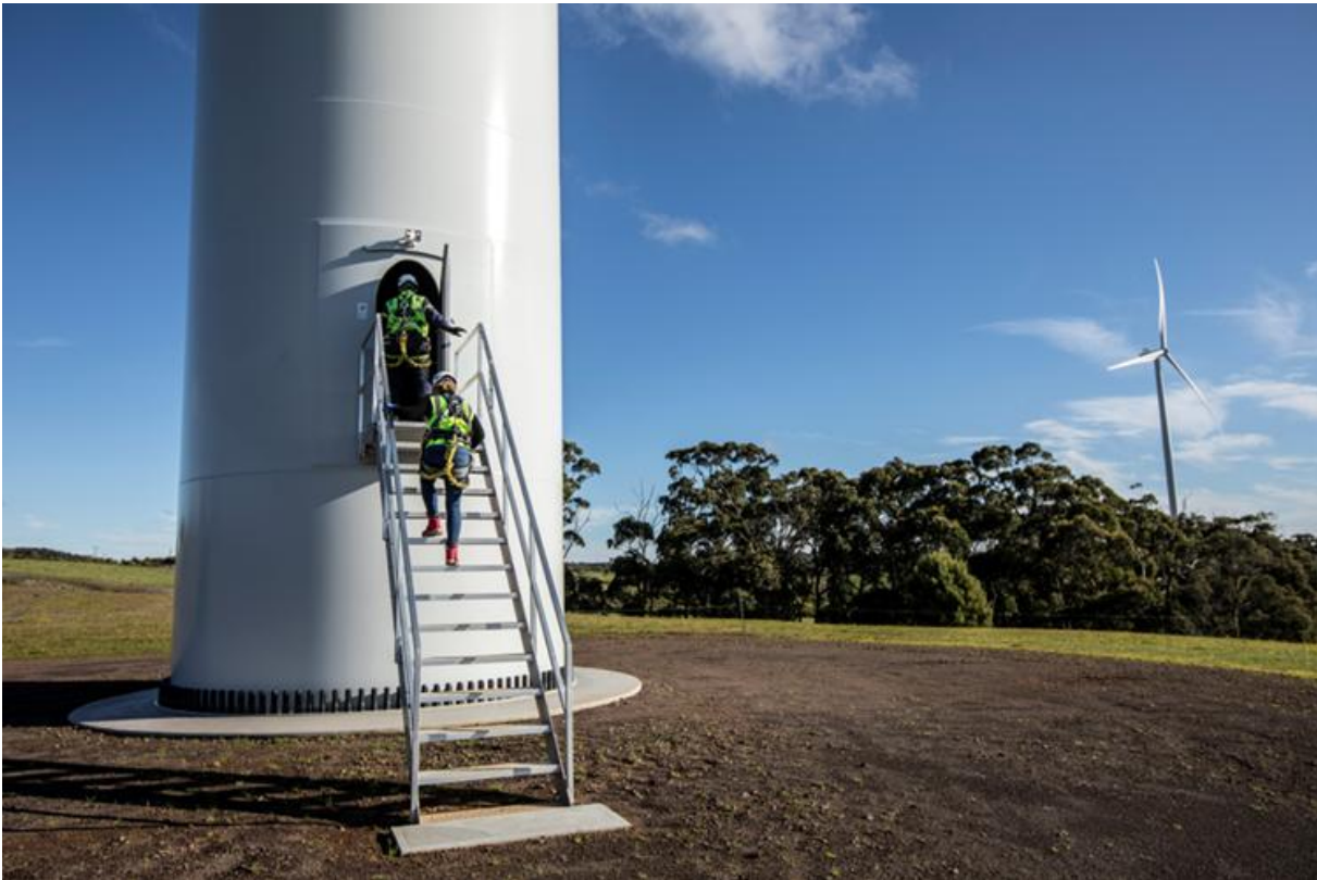
Photo 1.4 Typical WTG Hardstand Area
