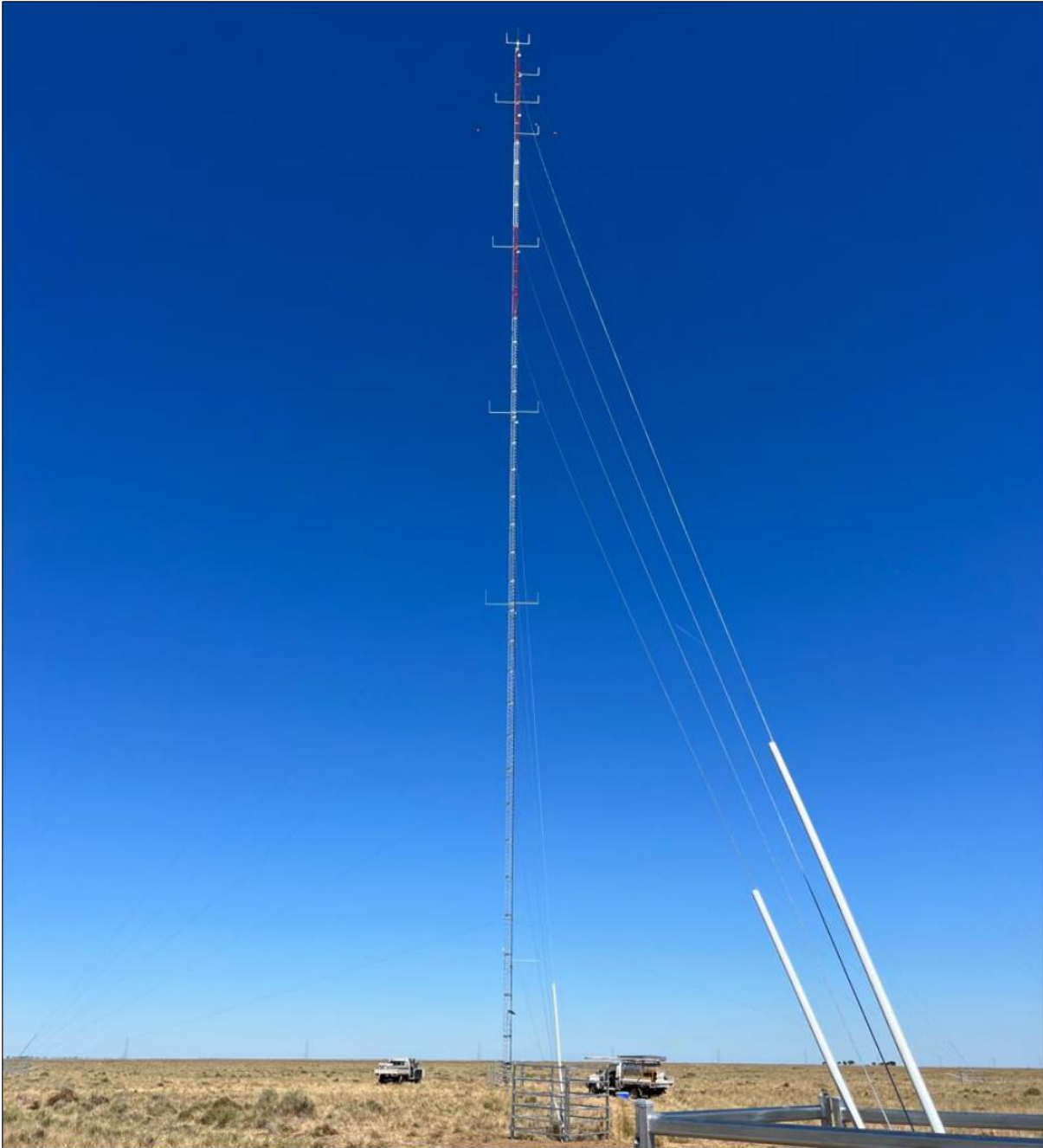
Photo 1.6 Typical Meteorological Mast
