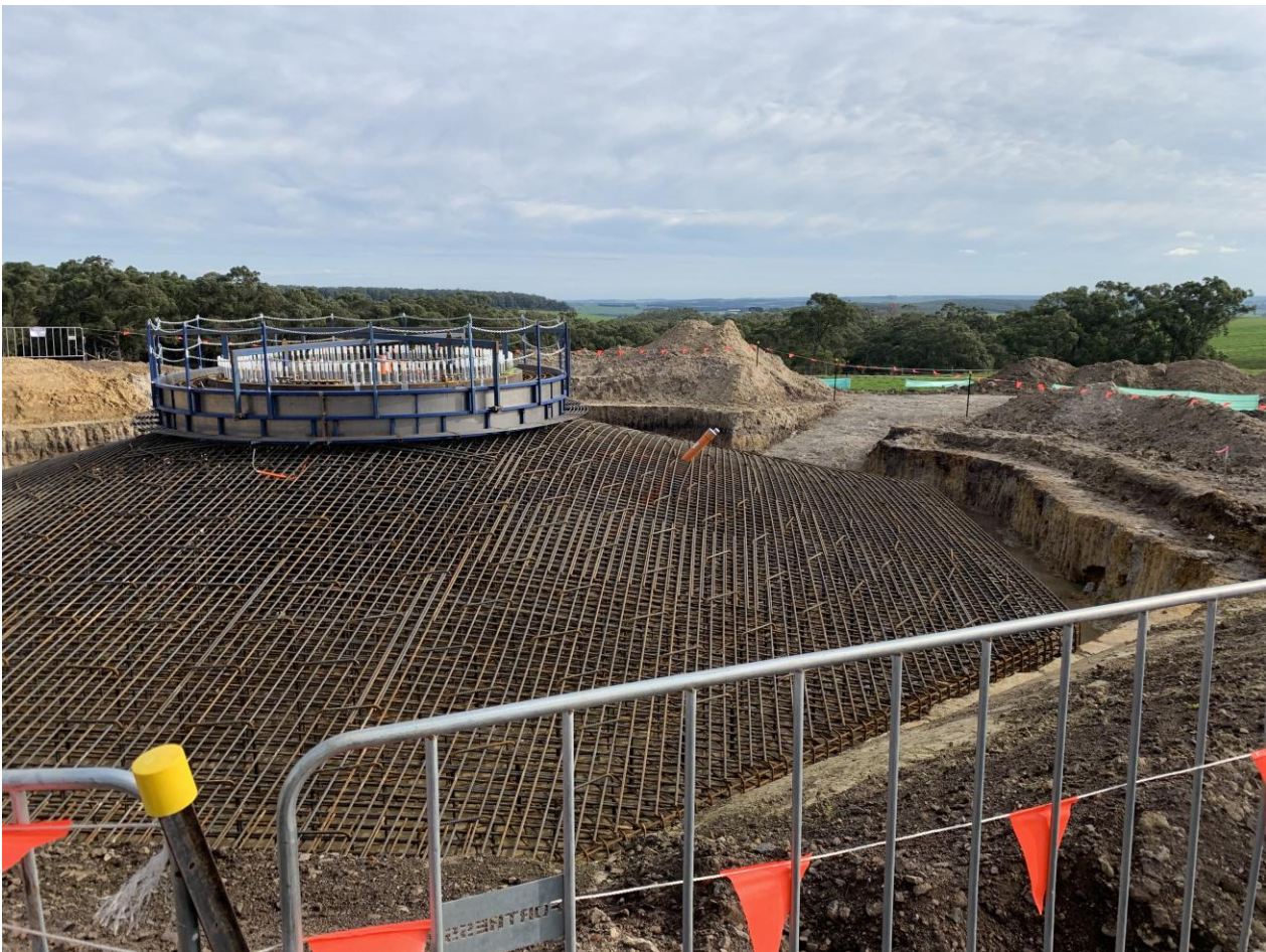
Photo 1.1 Typical WTG Foundation Under Construction
