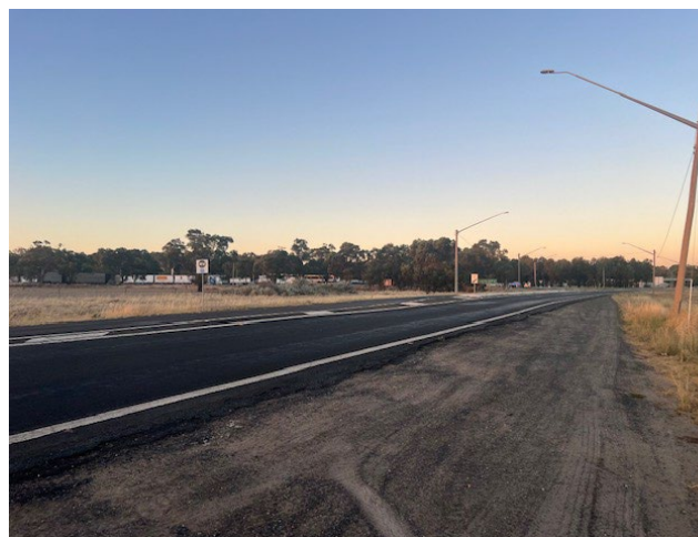
Photo 4.6 Eastern side of Off-Site Road Works Area along Cobb Highway Street
