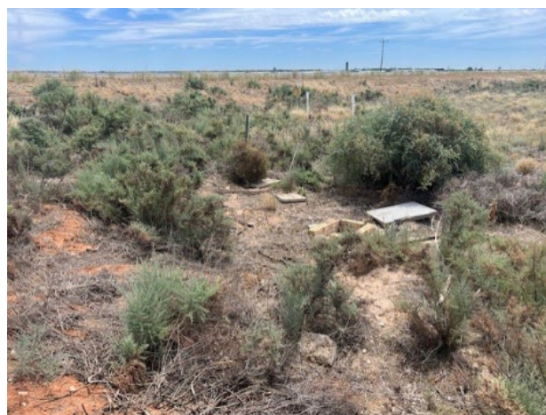
Photo 4.2 Northeastern side of Euston Off-Site Road Works Area
