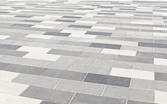
Public & Private domain: Concrete Unit paving
