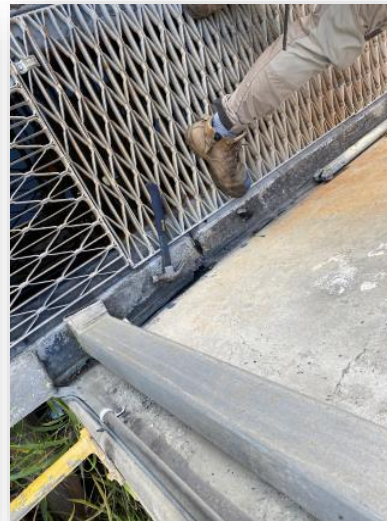
Example: Mastic sealant – Between pathway and wall of building
