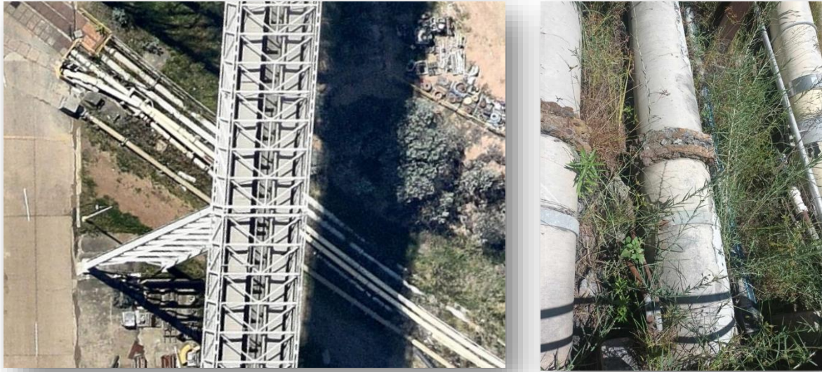
Example: Asbestos Cement Pipes – Ash & Dust Lines
