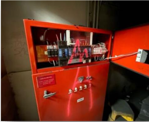
Example: Fuses in electrical board with friable fuse packing
