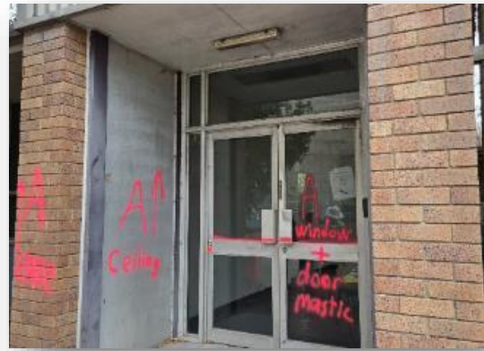
Example: Of windows and doors with mastic to windows
