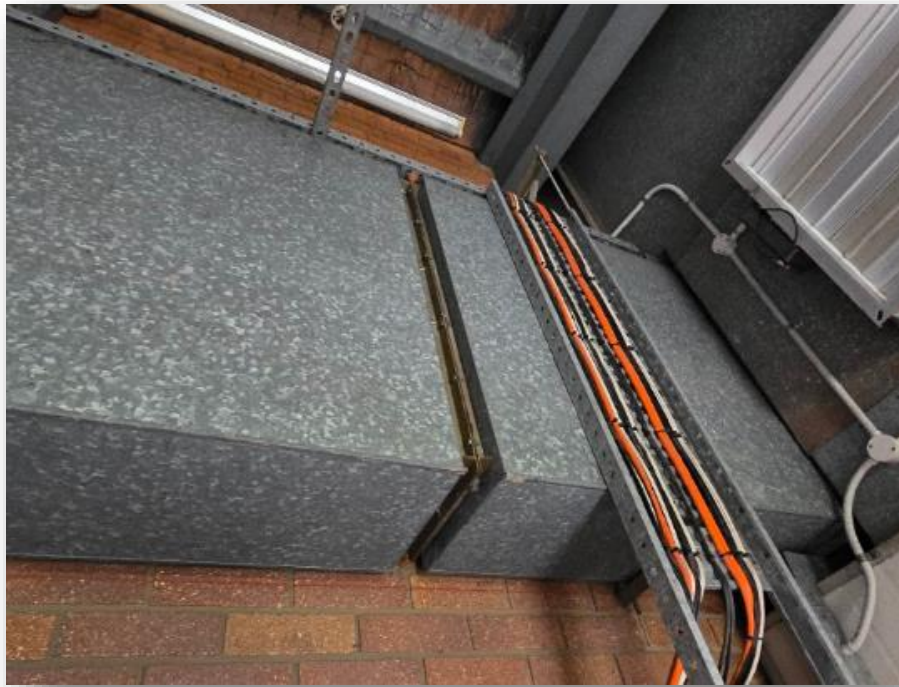
Example: Mastic at joins in ductwork
