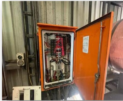
Example: Fuses in electrical board with friable fuse packing
