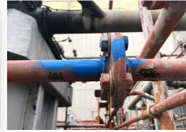
Pipework (202-16) – Non-Friable
