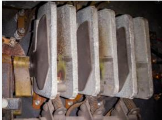
Example: Electrical arc shield within electrical box in transformer
