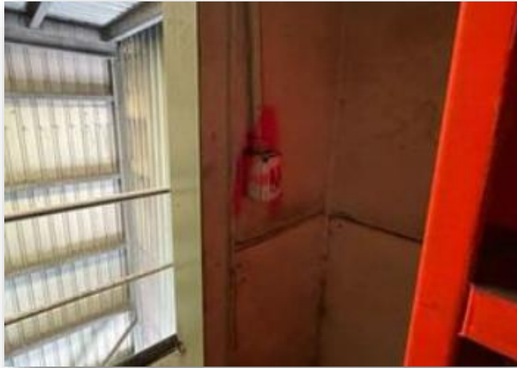
Example: Nilsen Switch with asbestos rope seal
