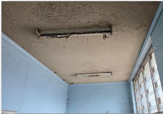
Example: Asbestos Containing Sprayed Vermiculite to ceiling
