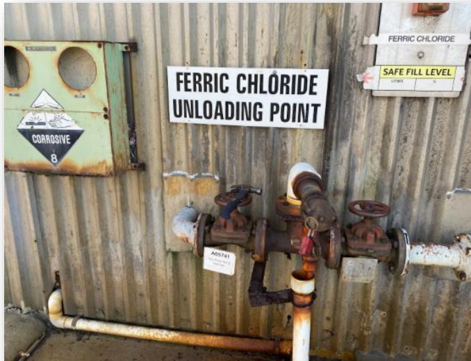
Example: Mastic sealant – around pipe penetration in wall
