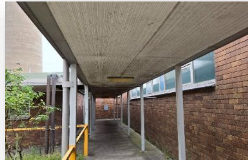
Example: Soffit of walkways
