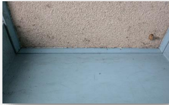
Example: Mastic sealant at corner of ceiling
