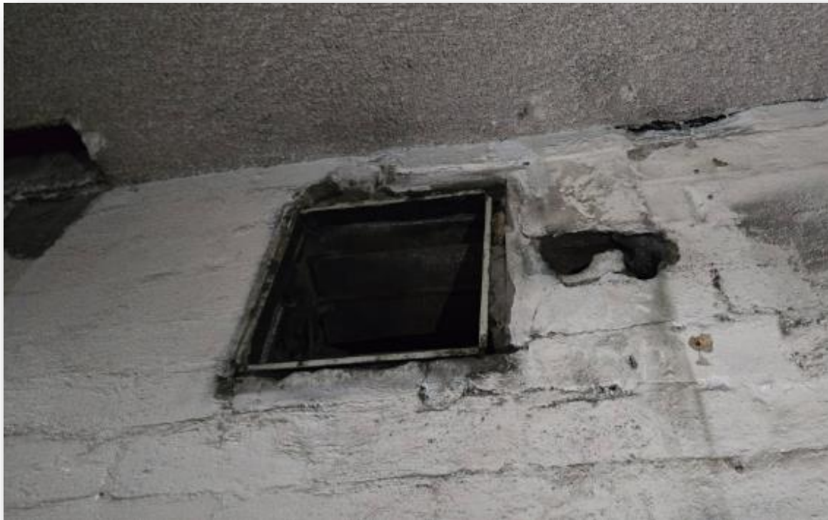
Example: Mastic sealant on the wall (opening edge)
