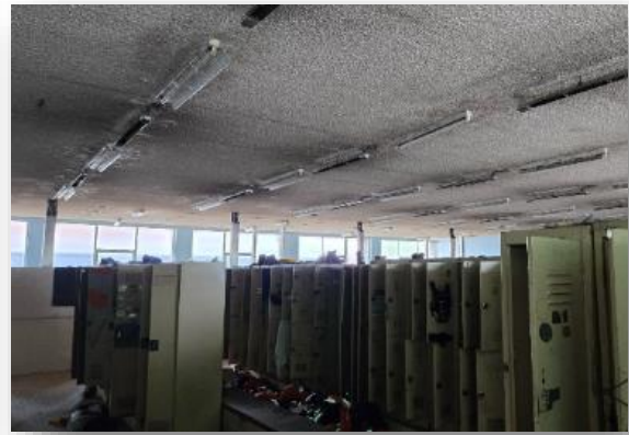
Example: Asbestos Containing Sprayed Vermiculite to ceiling
