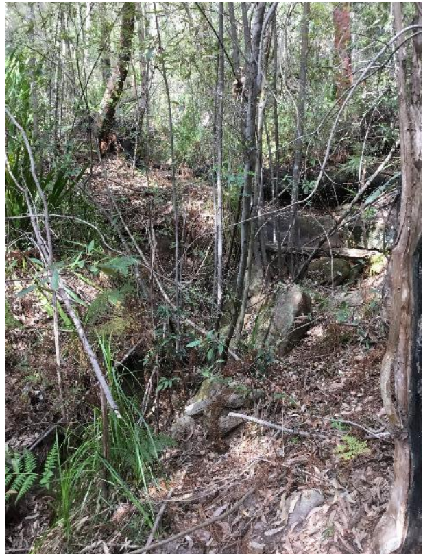
Photo S-East 1 (Upstream)
