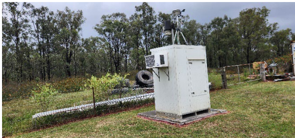
Monitoring station (TEOM) near mushroom composters (D4)
