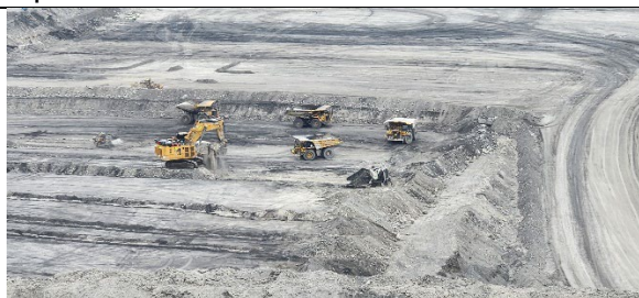
Earth moving plant in operation
