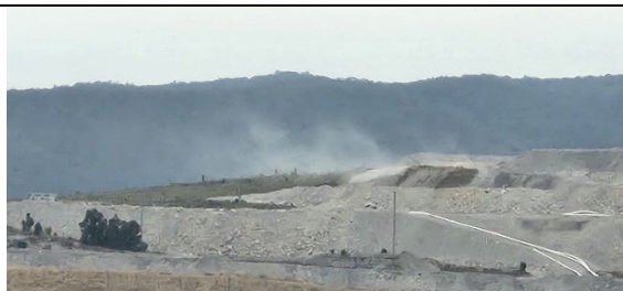
Dust plume visible during site walk
