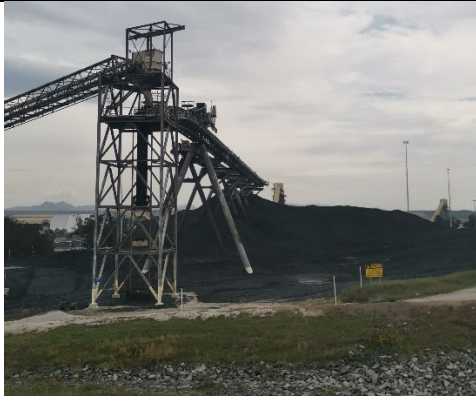
Coal stockpile - CHPP
