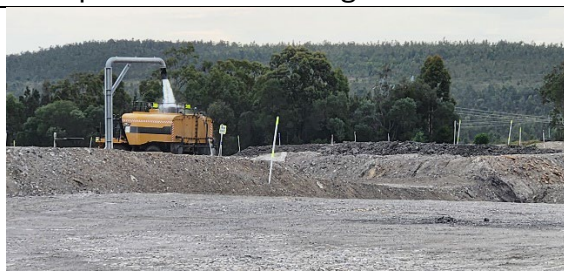
Water truck for dust management being filled
