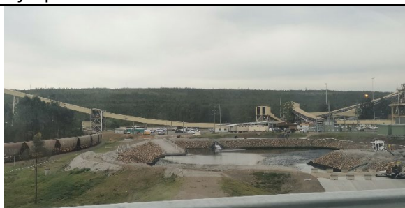
Rail line, pond and Coal Handling and Processing Plant
