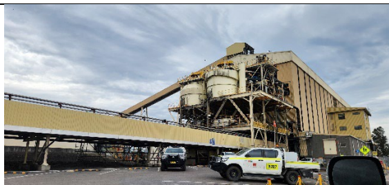
Working plant area
