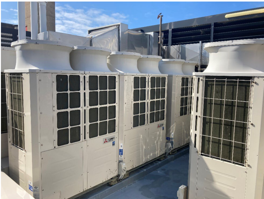
Rooftop HVAC area
