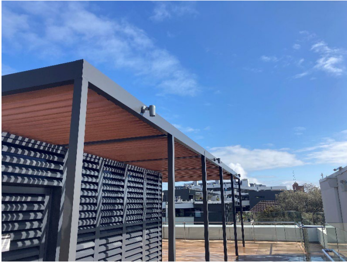
Exterior of rooftop HVAC area, noting downward facing lights
