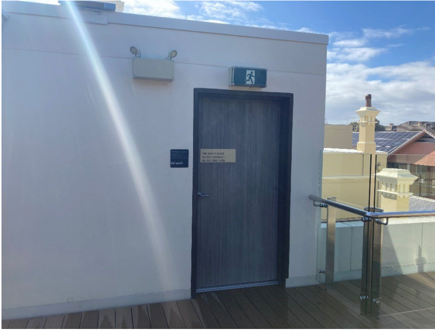
Rooftop emergency exit
