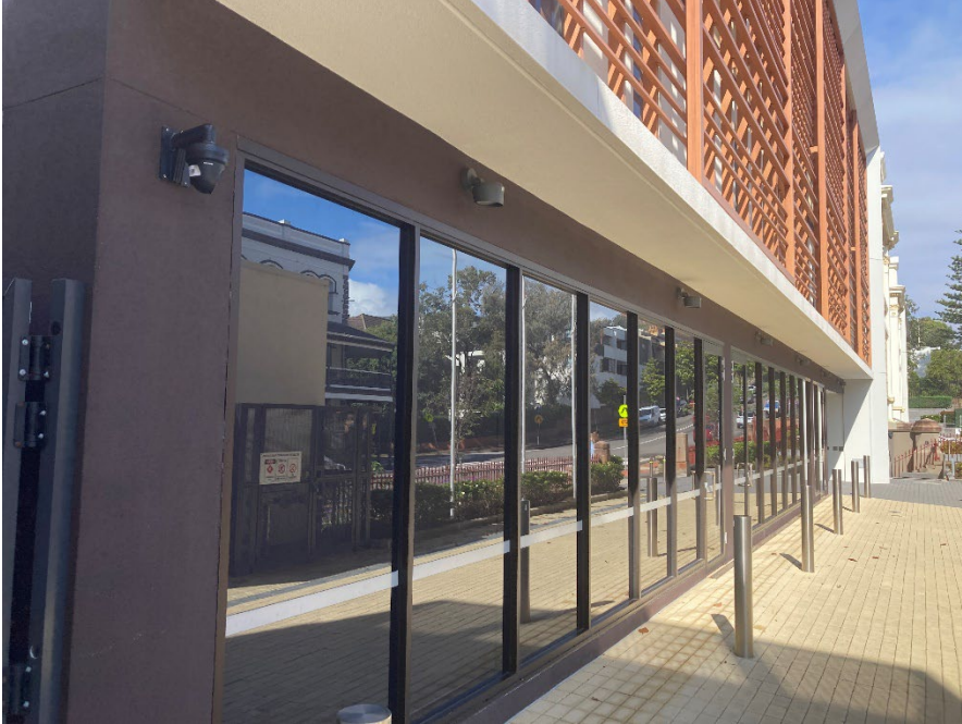
Front façade of building and service area
