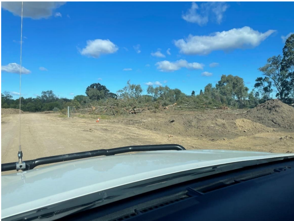
Plate 10 Cleared vegetation stockpiled within Area 2, Stage 2
