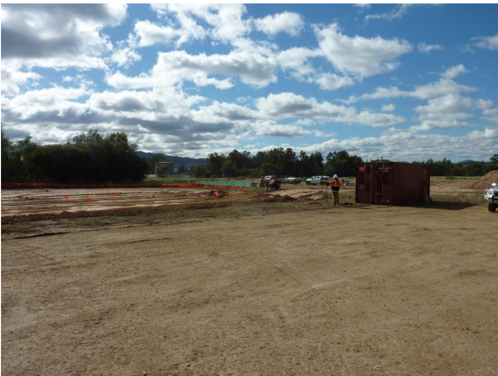
Plate 7 Sediment fencing within the Stage 2 area, including around stockpile
