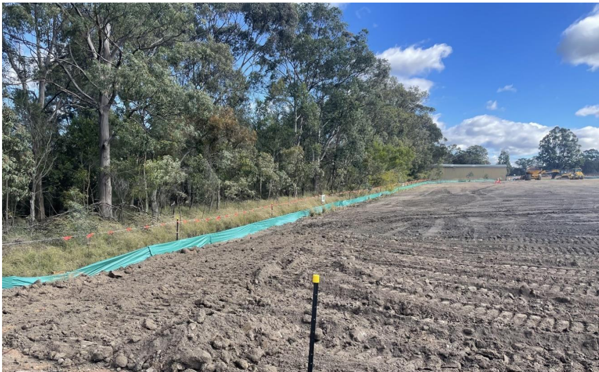
Plate 2 Area 1, Stage 2 sediment fencing and disturbance boundary delineation
