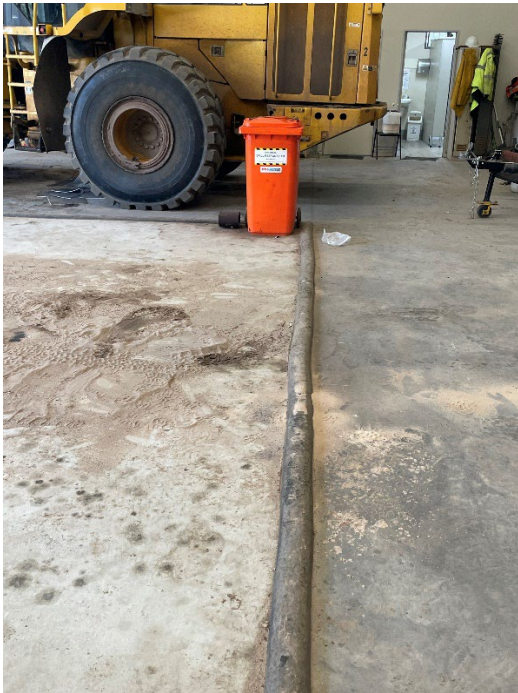
Bunded workshop area
