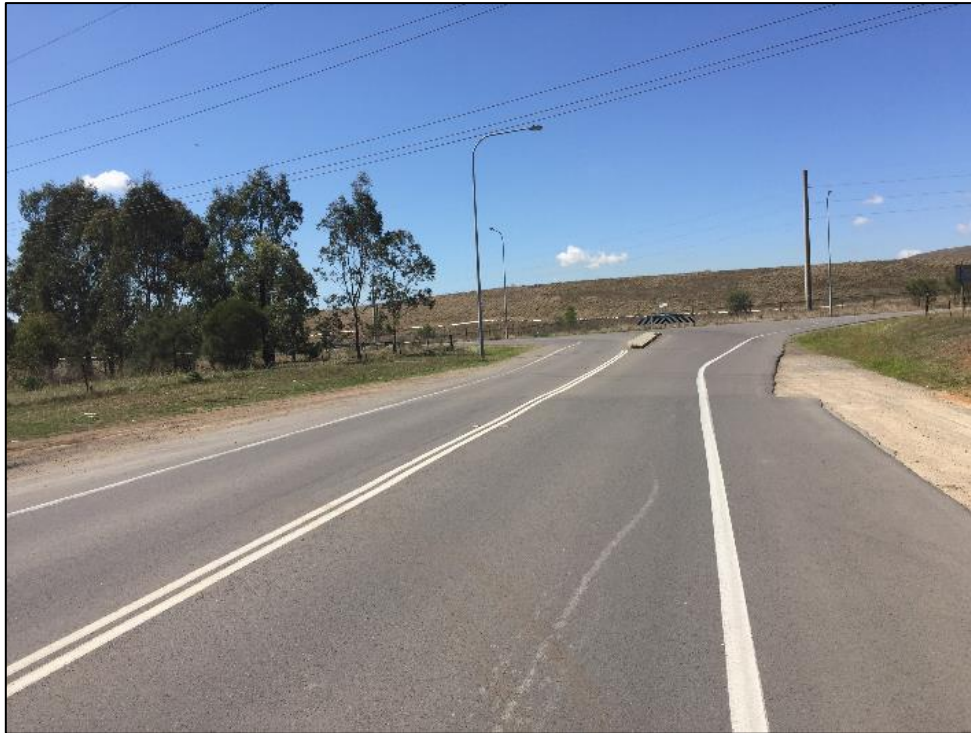
Figure 5 Bengalla Road looking south towards Denman Road
