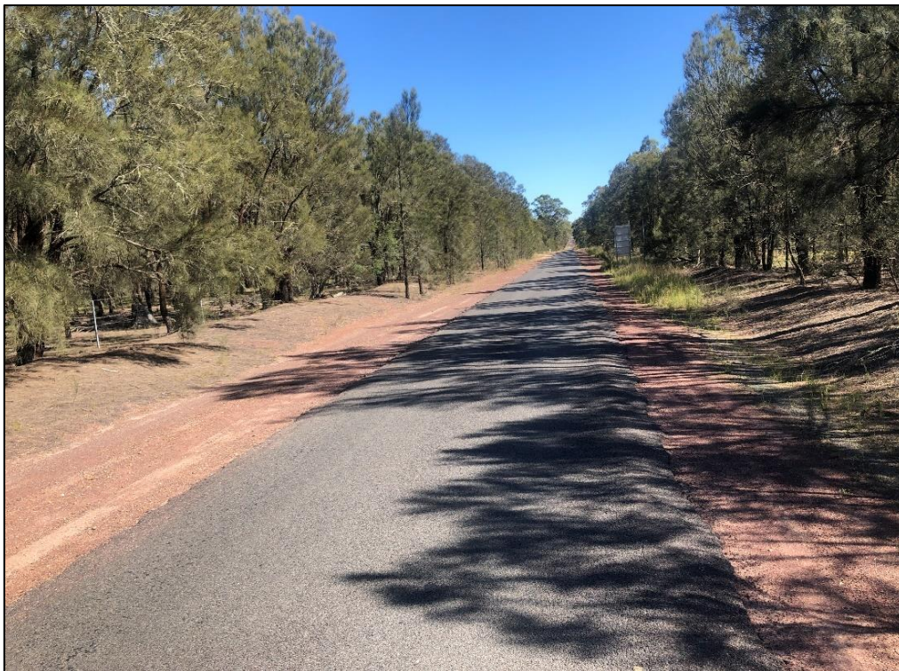
Figure 9 Former Wybong Post Office Road Looking West
