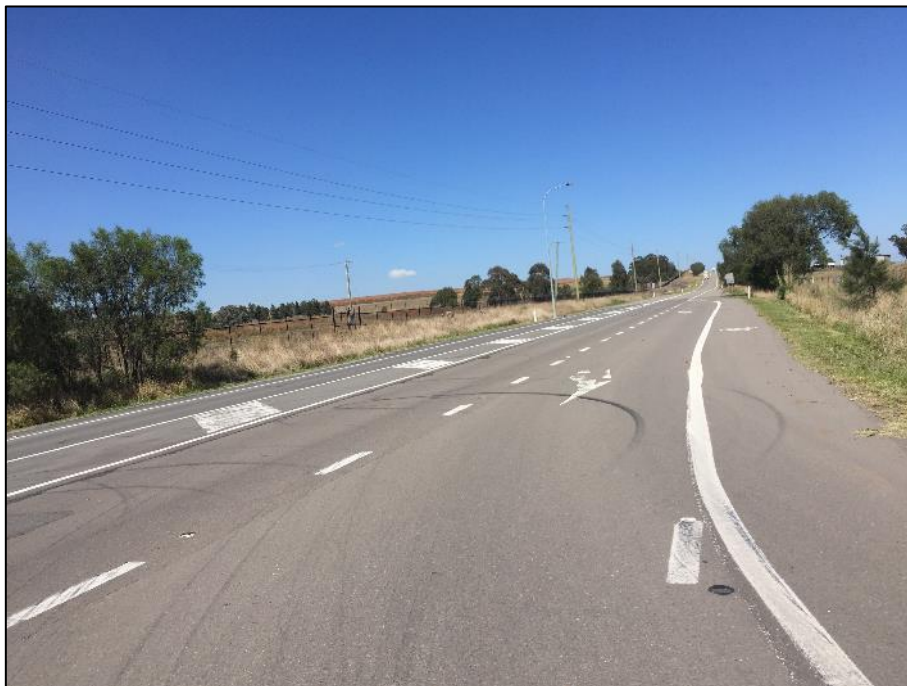
Figure 7 Denman Road looking west from Bengalla Road
