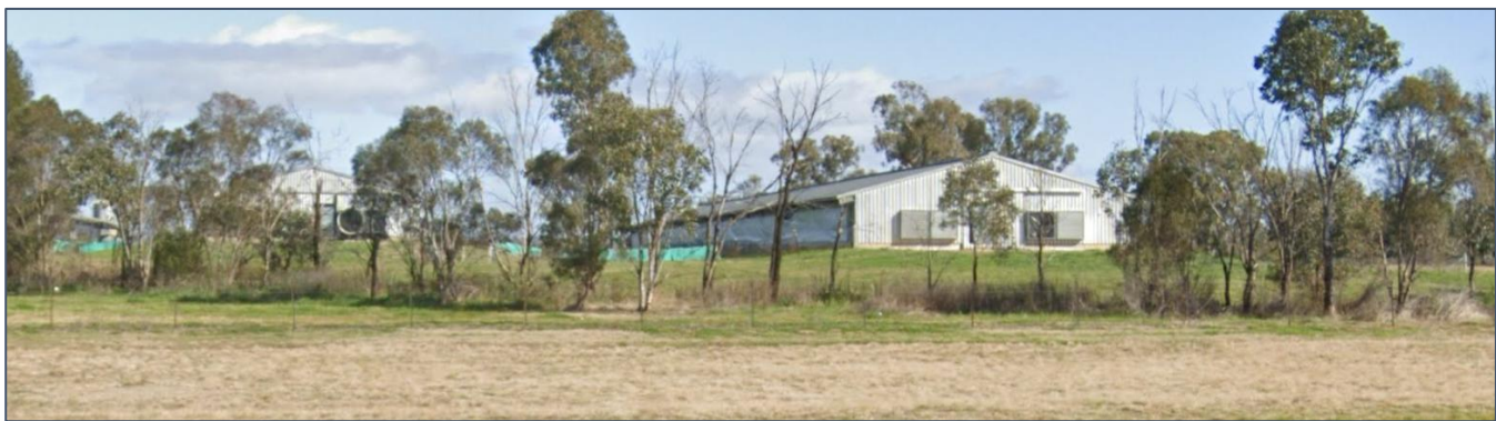
Figure 33: Adjoining Bowlers Lane 1 Broiler Farm (Bowlers Lane)
