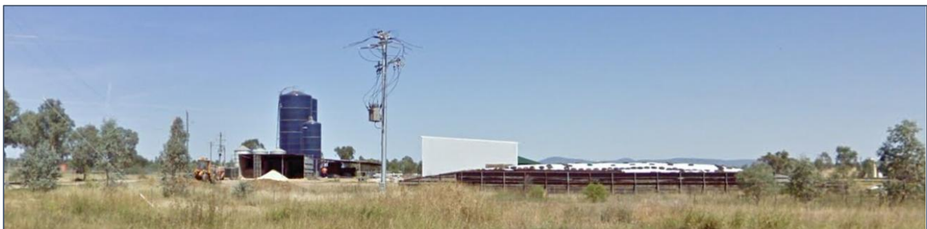
Figure 34: Adjoining Dairy (Wallamore Road)
