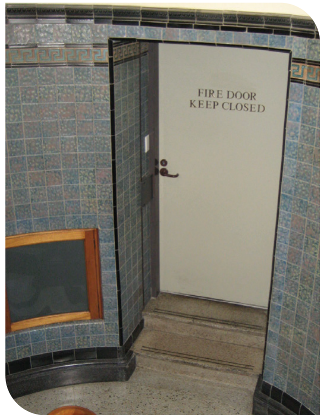
Stairwell with 1960s openings.
