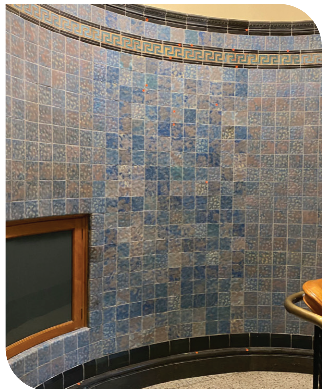
Infilled wall with salvaged and new.
