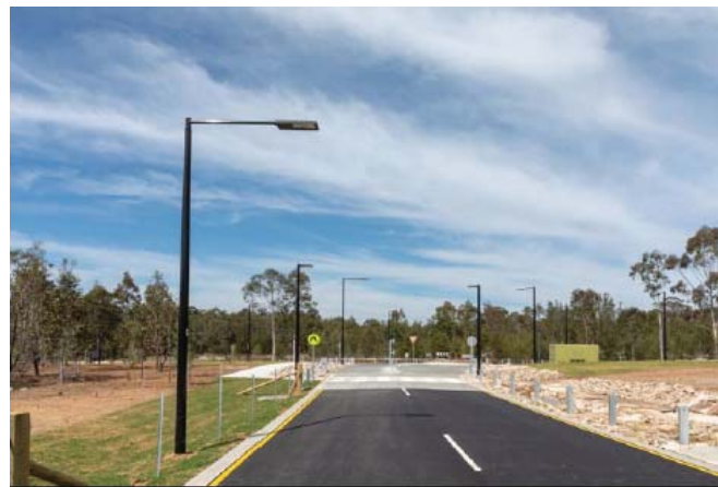
Street Lighting Pole (Source: WSPT Design Manual)
