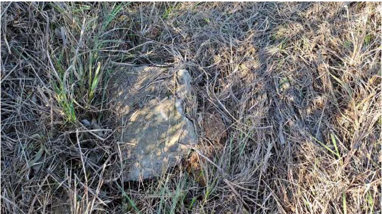
Image 6.8.4 View of the concrete block, in the northeast portion of the site
