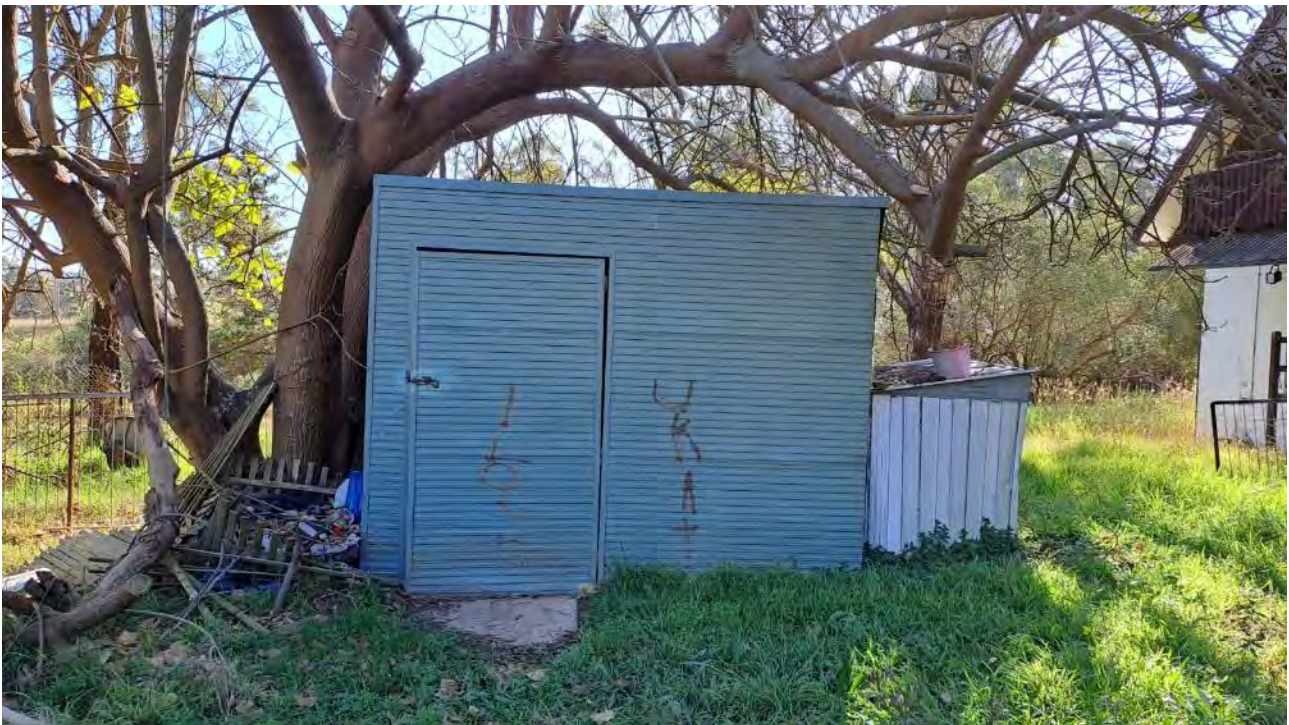
Image 6.2.2 View of single storey metal storage shed (shed 1) in the backyard of the house, facing north
