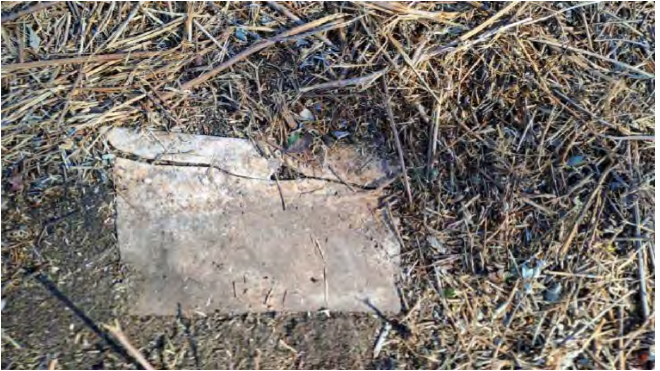
ACM sheet, located to the immediate north of the Residential Dwelling.
