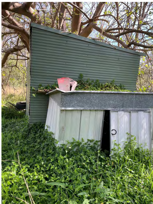
Image 6: Storage Shed located in the south-eastern portion of the site to the west of the Residential Dwelling.
