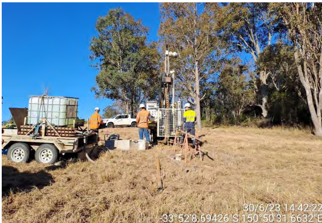
Image 8.1.1 View of sampling work at BH05, facing east
