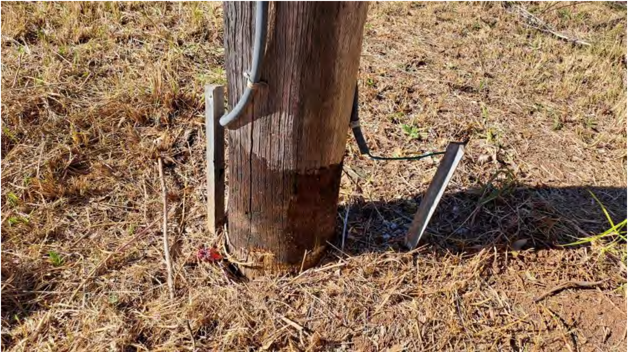
Image 6.2.5 View of potentially termite treated power pole within the southeast portion of the site
