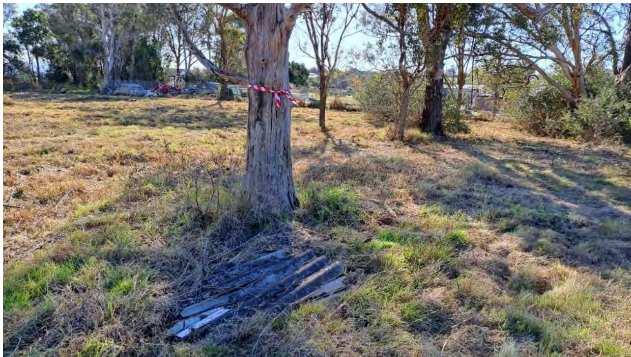
Image 6.10.2 View of corrugated ACM roofing sheets, in the northeast portion of the site
