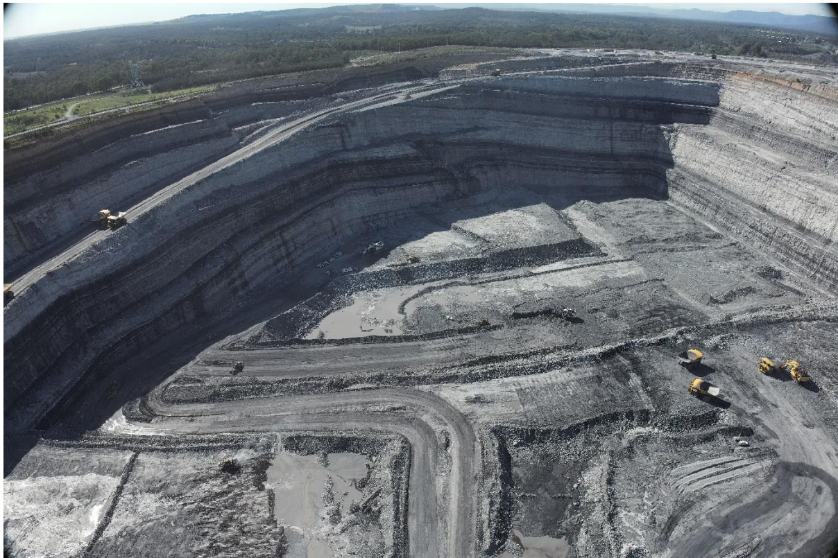
Figure 4-1 United Open Cut operations in December 2023
