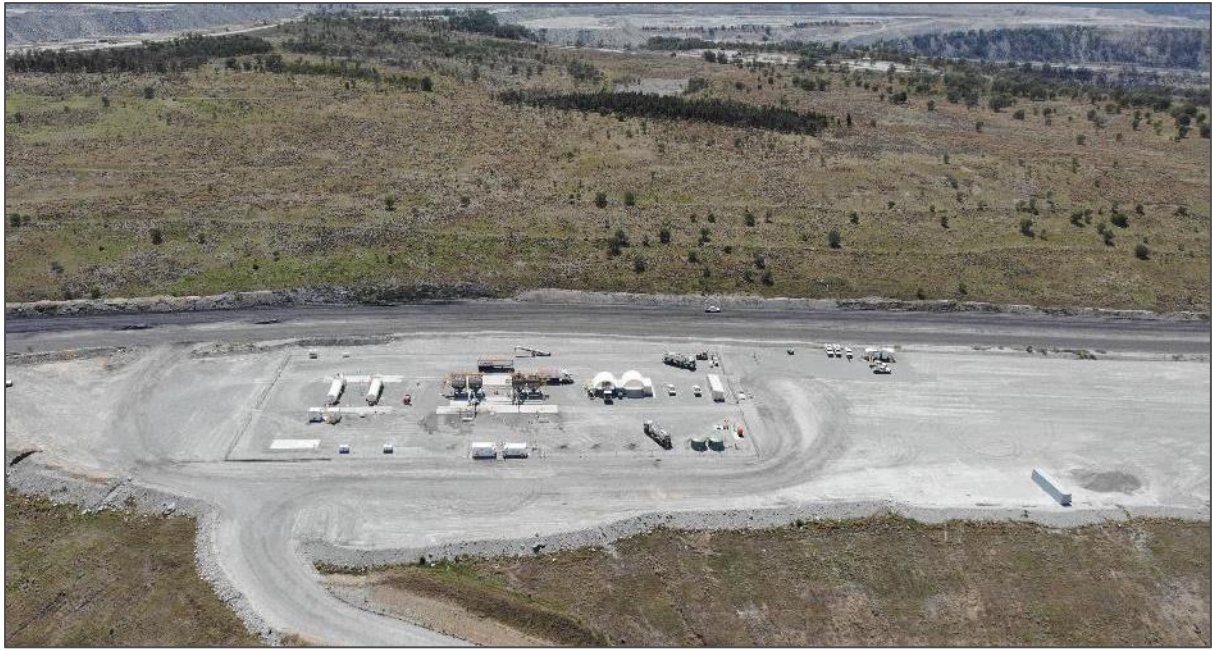
Figure 4-2 Reload and magazine area constructed
