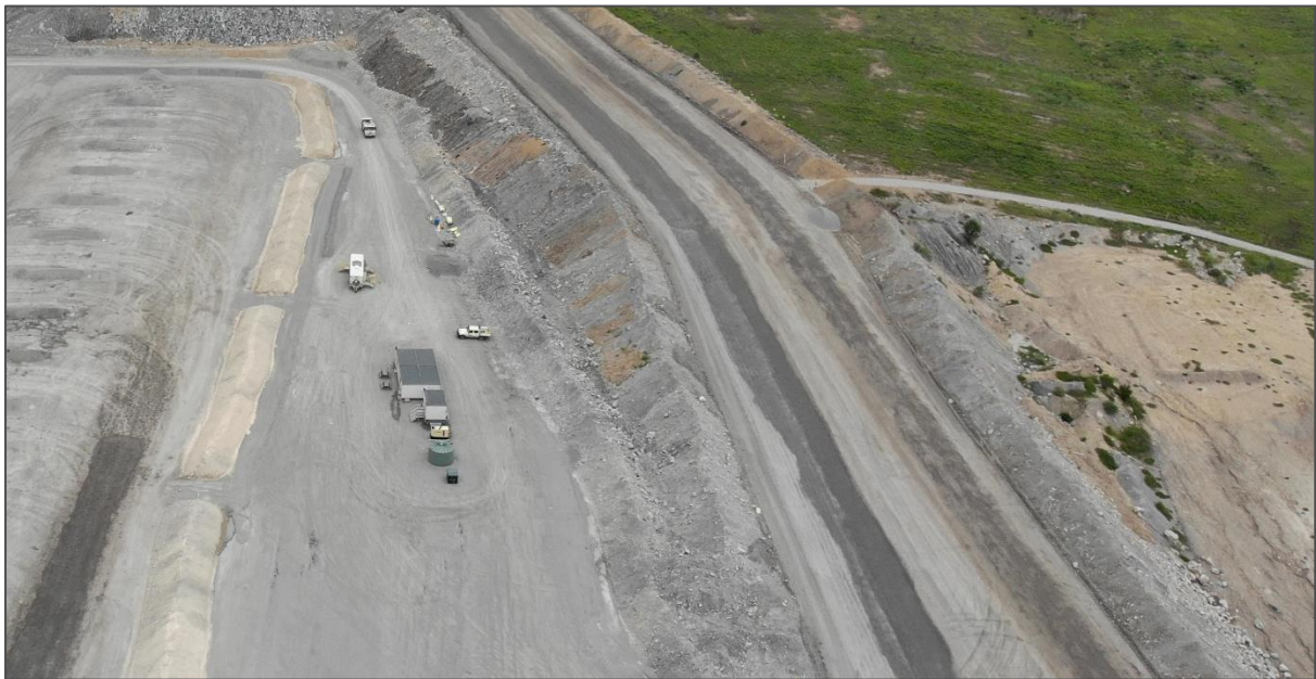
Figure 4-3 Montrose crib hut constructed
