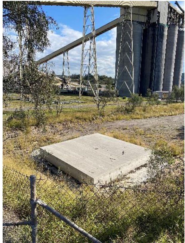
Photograph F.53 RUM shaft closure and rehabilitation
