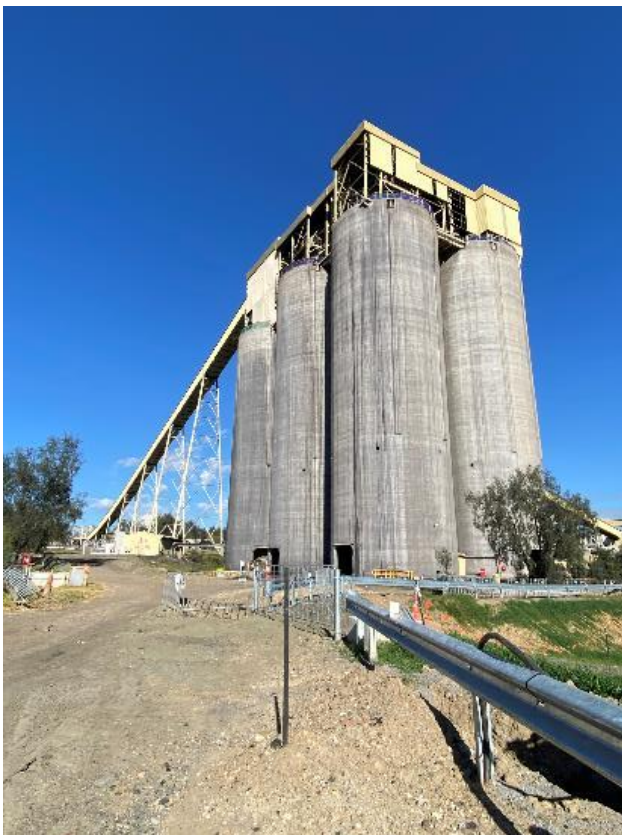
Photograph F.26 Replacing transfer chute cladding
