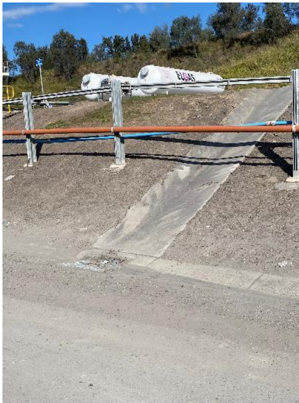
Photograph F.84 Surface water management
