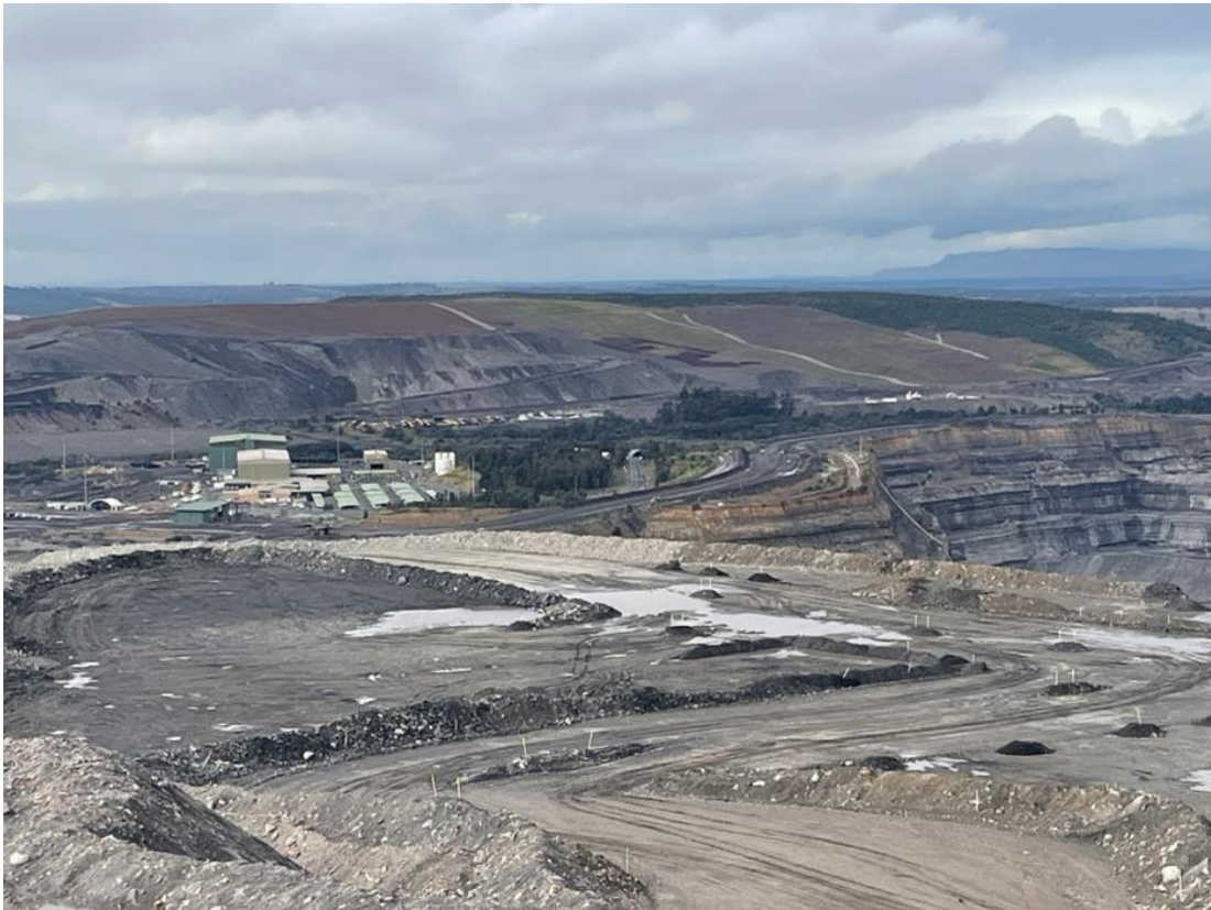
Photograph F.95 Active mining areas and different stages of rehabilitation on the Eastern Emplacement Area (EEA) (note rock lined geomorphic drainage lines)
