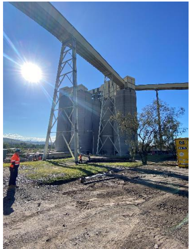
Photograph F.43 Coal storage bins
