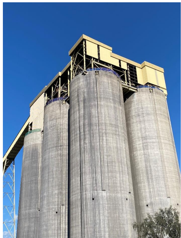
Photograph F.27 Replacing transfer chute cladding
