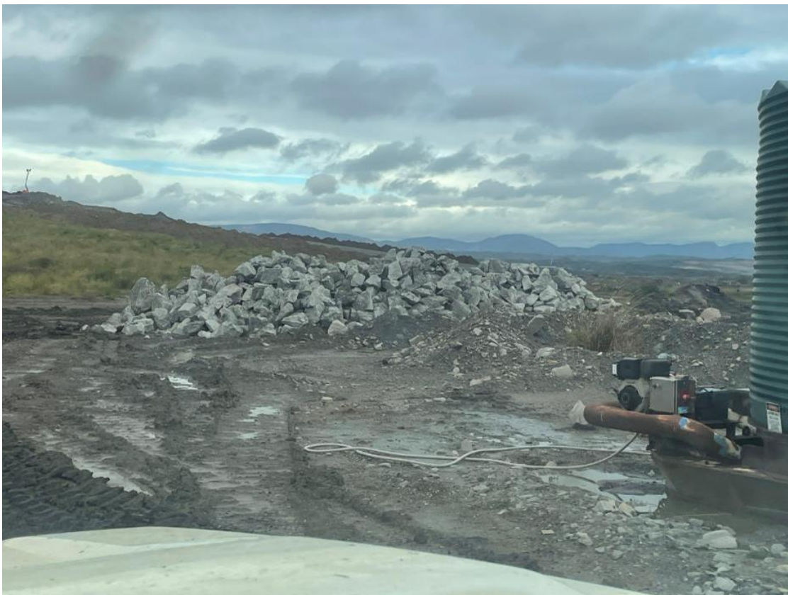
Photograph F.98 Rock RipRap being saved for use in geomorphic drainage lines
