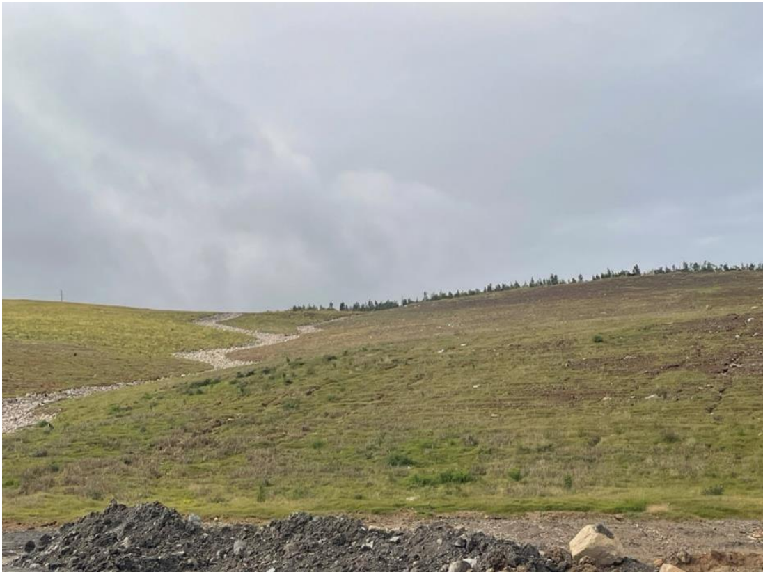
Photograph F.105 Recent rehabilitation with geomorphic landform and drainage, note some rill erosion to be addressed in maintenance program
