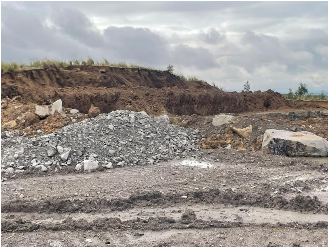
Photograph F.97 Active topsoil stockpile on the EEA being used to spread over prepped landform
