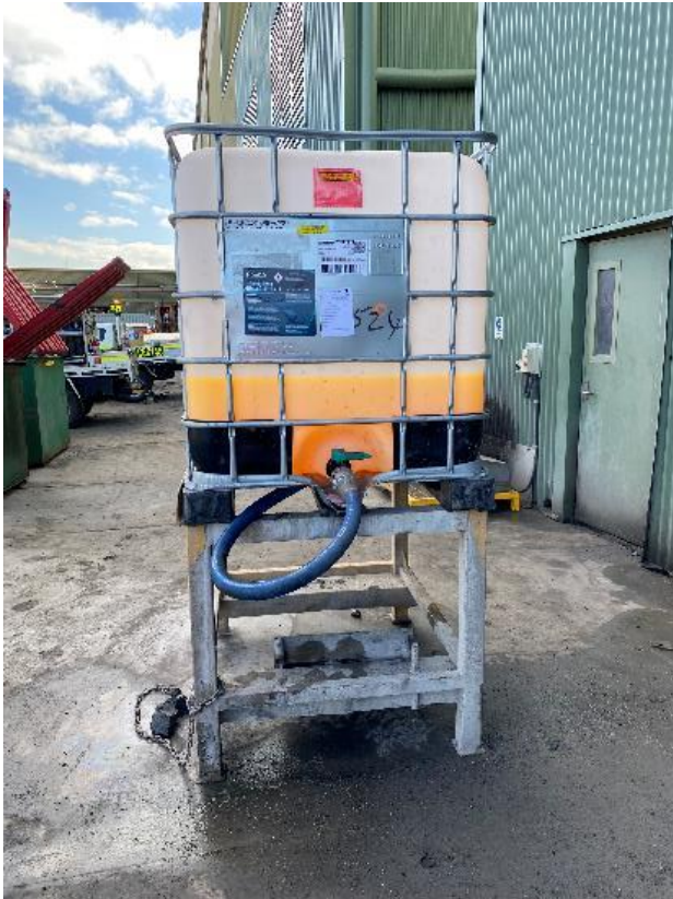
Photograph F.73 Hydrocarbon storage
