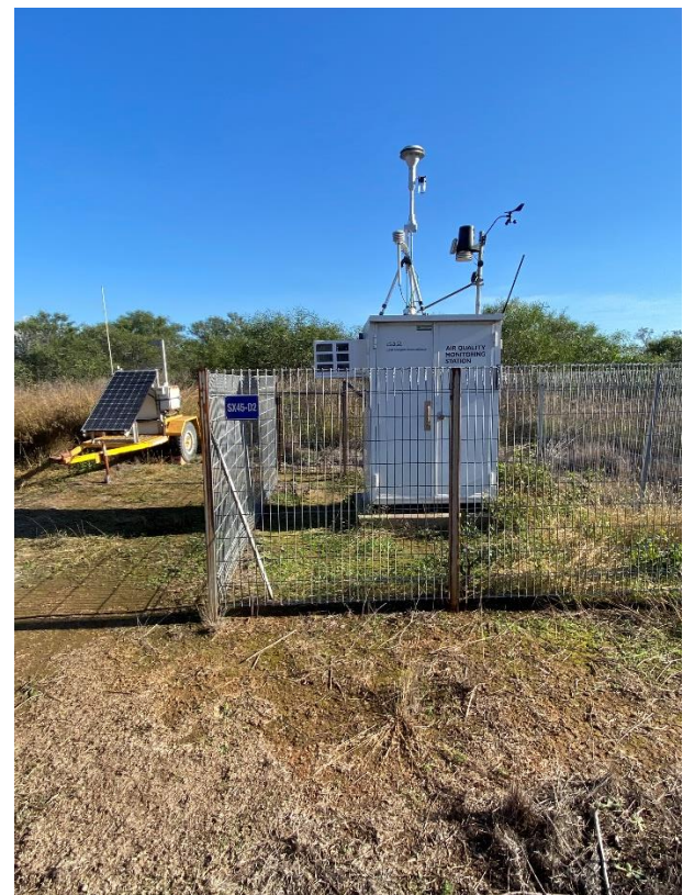
Photograph F.17 Air quality monitoring station
