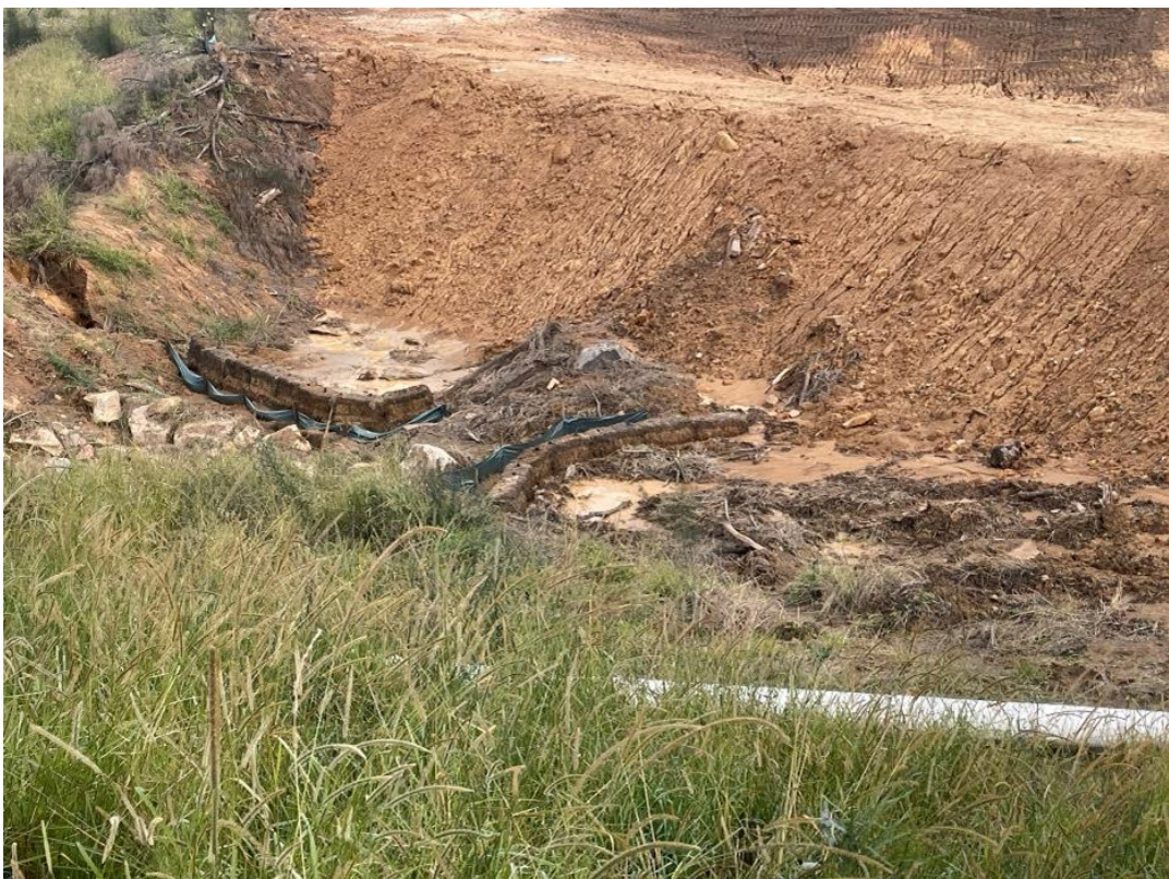
Photograph F.106 Temporary ESC measures adjacent access road to minimise sediment laden water flowing to sedimentation pond
