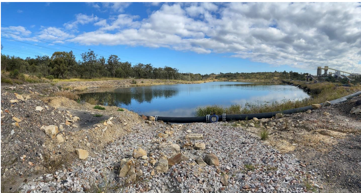
Photograph F.54 Highway Dam
