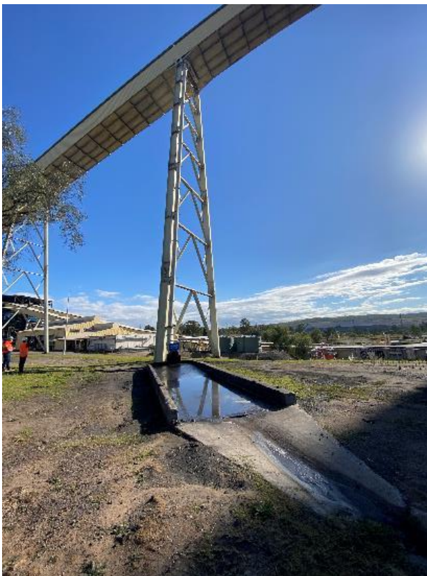
Photograph F.46 CHPP water runoff
