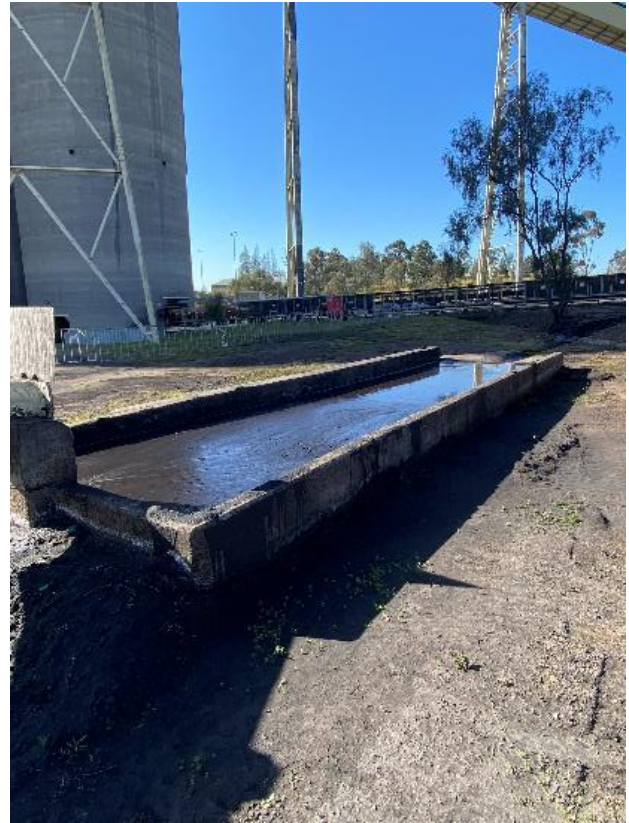
Photograph F.45 CHPP water runoff
