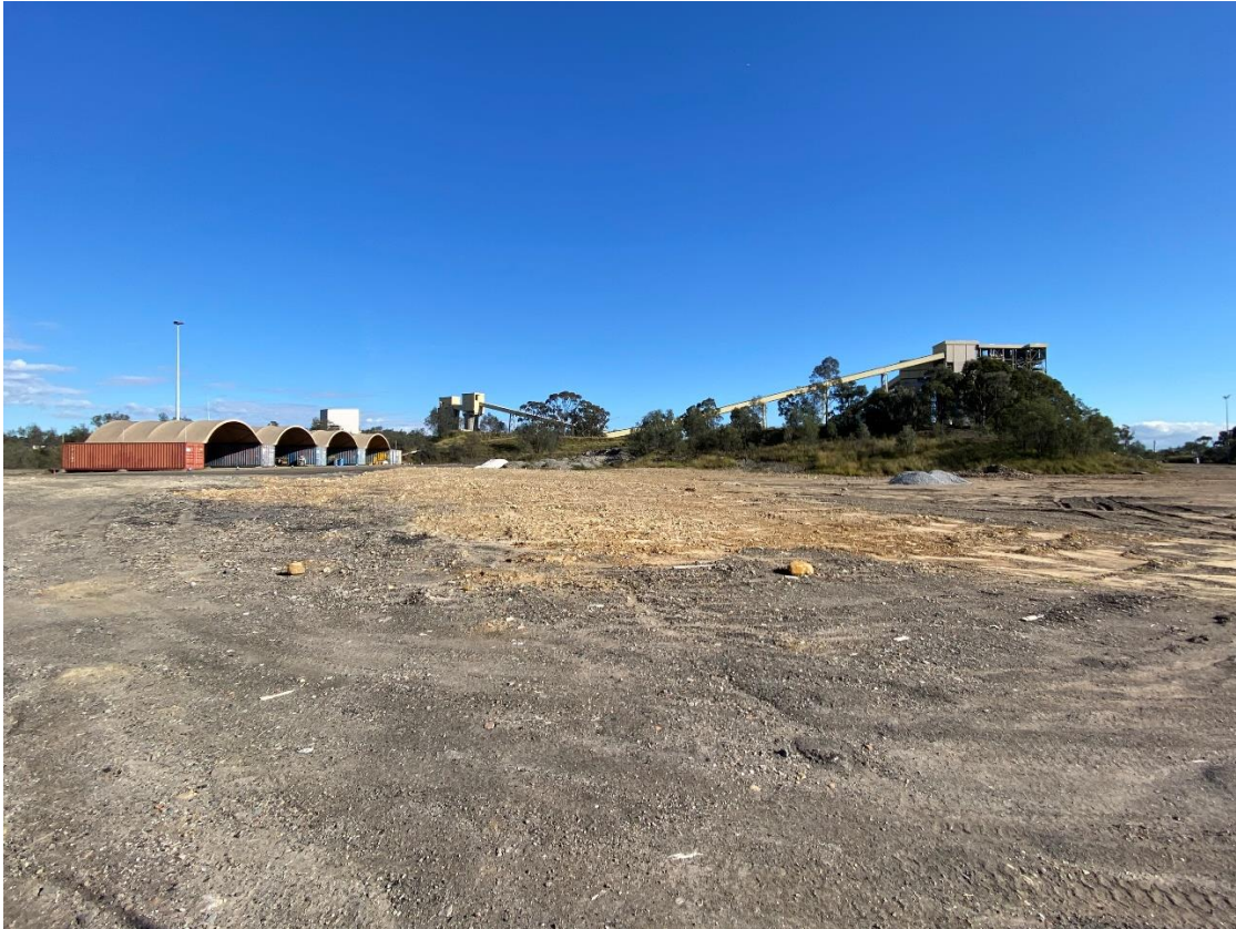
Photograph F.25 Demolition area at RUM
