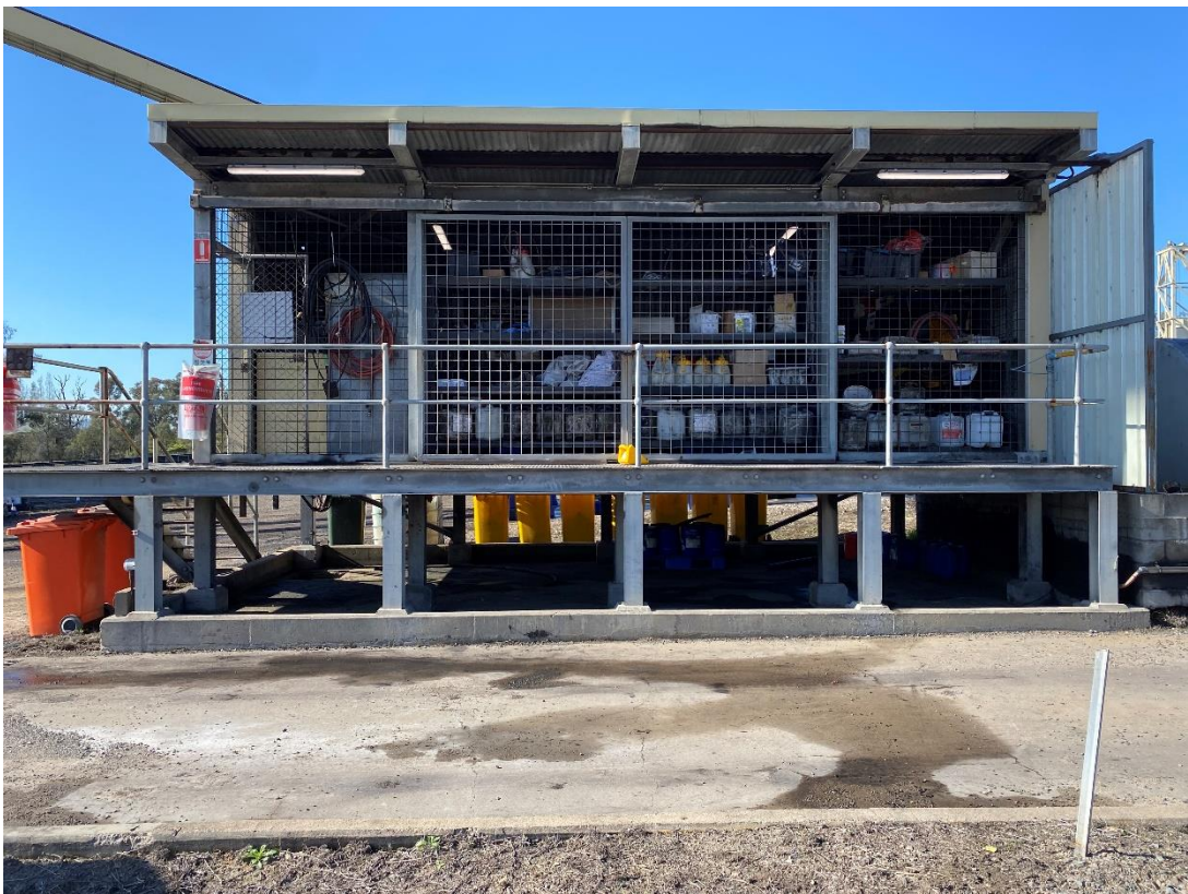
Photograph F.29 Hydrocarbon storage
