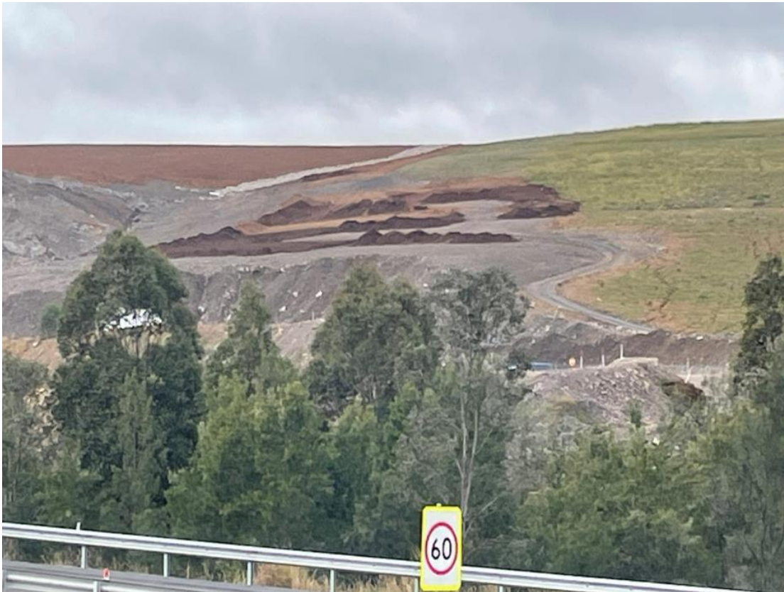
Photograph F.107 Topsoil being placed on final shaped landform with varying stages of rehabilitation adjacent
