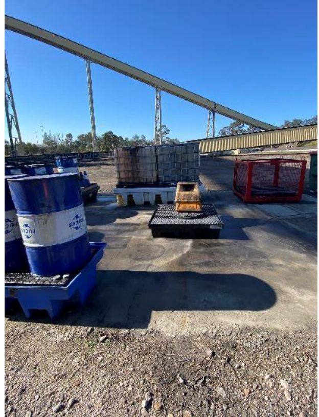
Photograph F.37 Hydrocarbon storage
