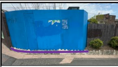
Sandstone edging to be protected during construction
