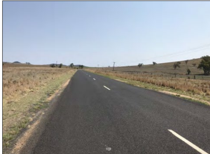
Figure 4-1 View along Bruxner Way in the vicinity of the Project Site (Source: TIA, 2020)
