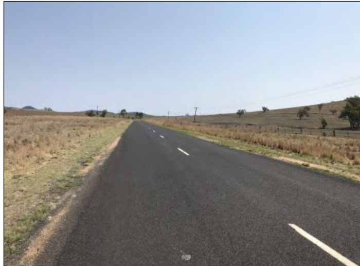
Figure 4-3 View along Bruxner Way in the vicinity of the Project Site (Source: TIA, 2020)
