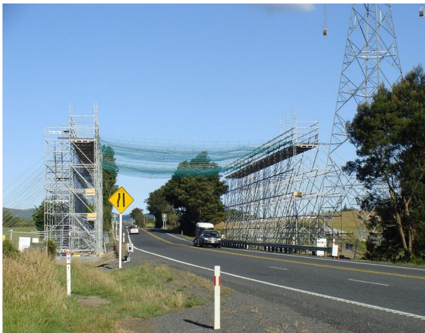
Figure 4-2: Example of a semi-permanent hurdle arrangement with safety netting. Indicative only.
