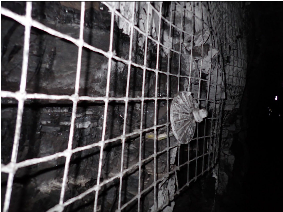
Figure 5: Rib support in 401 panel showing gloving of resin and unencapsulated bolt.
