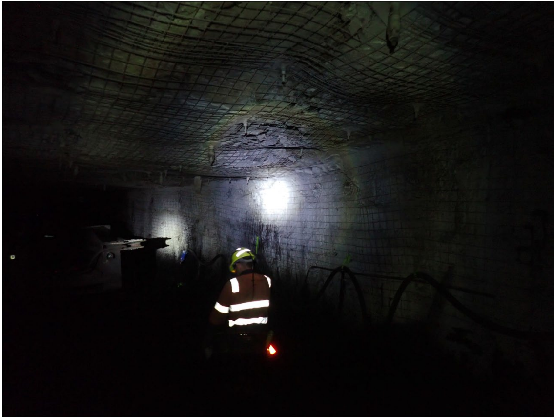
Figure 6: Fault observed in 401 panel leading into intersection showing roof deformation with square ribs at 200m DOC.
