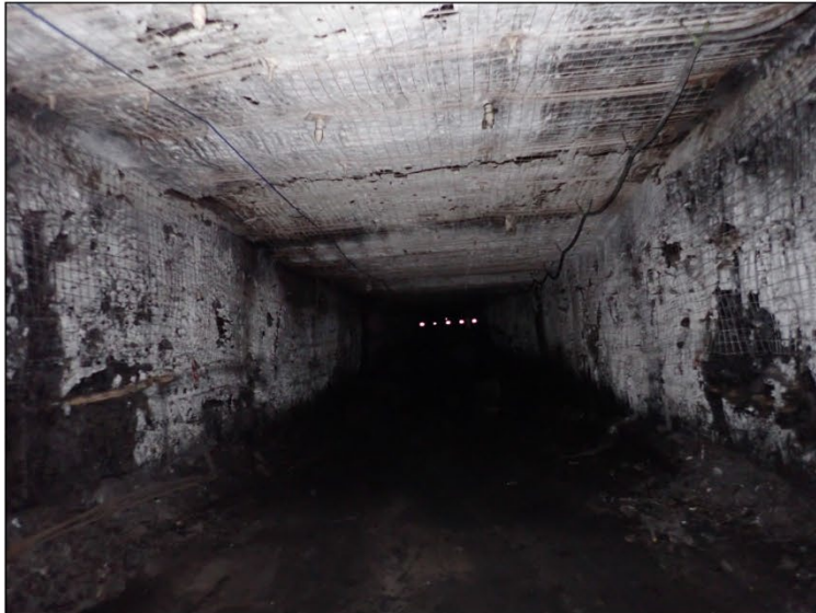
b) D-E HDG 12CT 120m DOC (20m out from under the cliff line).
