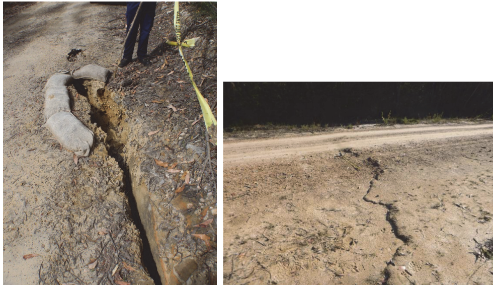
Fig. 6.2 Impacts along the unsealed roads and tracks above LW6 in Area 3A (left side) and above LW11 in Area 3B (right side) (Source: IMC)
