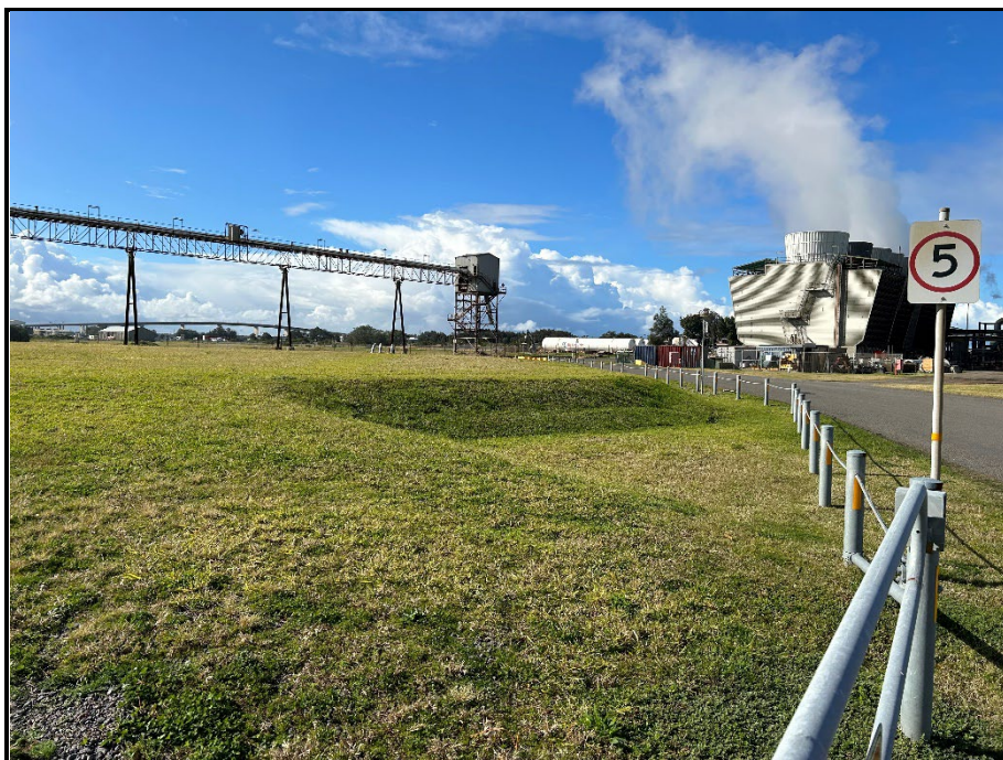
Photo 10: Containment cell looking northeast.
