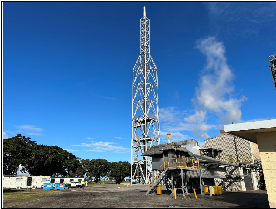
Photo 9: Replacement NAP1 stack.
