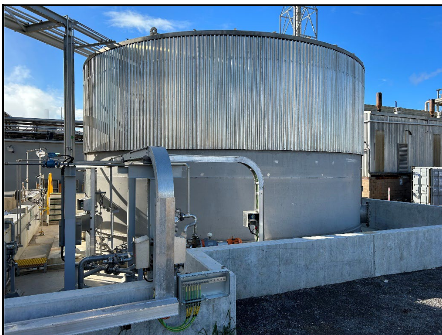
Photo 8: New effluent tank to replace pond with single liner.
