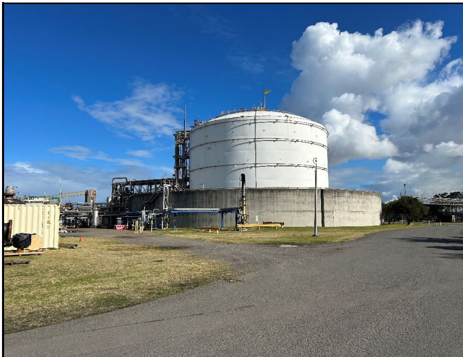
Photo 2: Ammonia storage tank within concrete bund.
