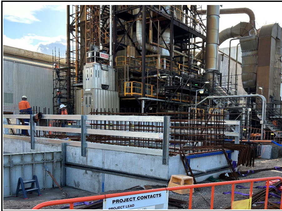
Photo 5: Scrubber under construction (Phase 8) at ammonium nitrate plant AN1.
