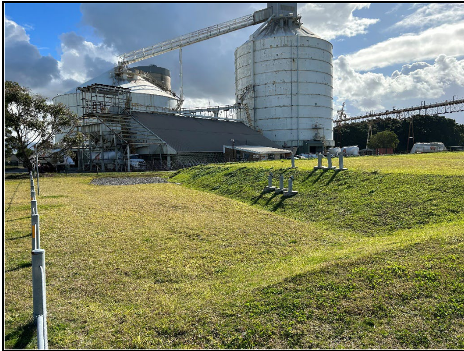
Photo 11: Containment cell looking west with fence (left), surface water catchment in background and set of monitoring wells either side of cut-off wall (centre).
