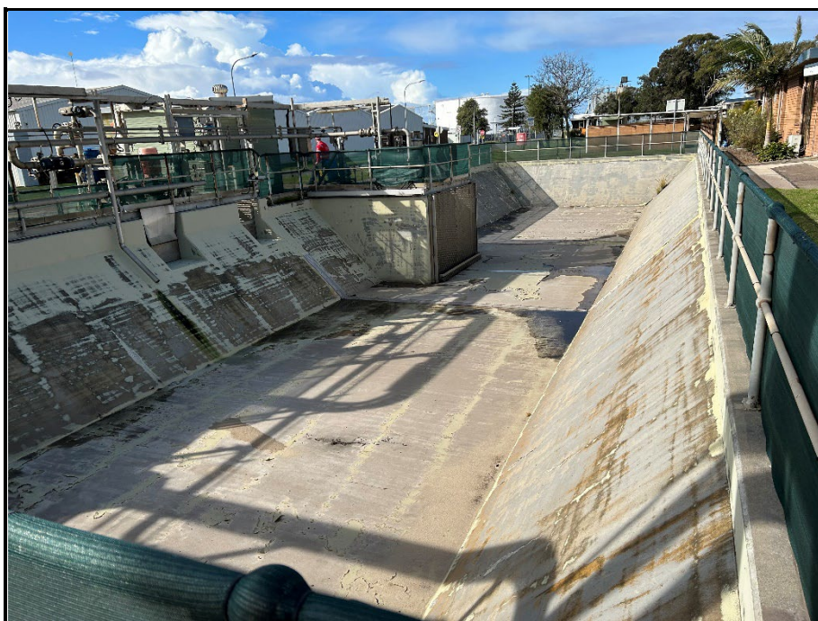
Photo 4: Effluent diversion basin.
