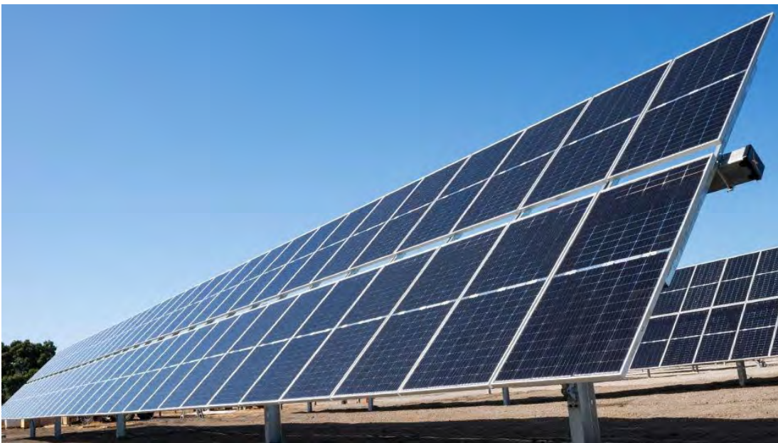
Plate 2.1 Example of a PV module layout (2 in portrait or 2P configuration)
