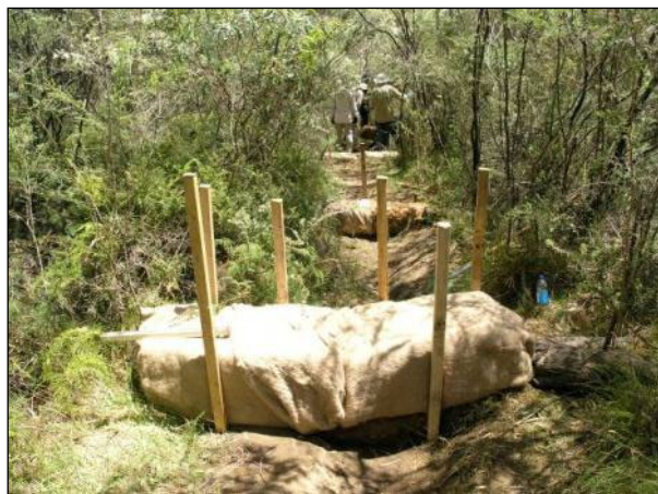
Figure 6-5 Small coir log dams with fibre matting
