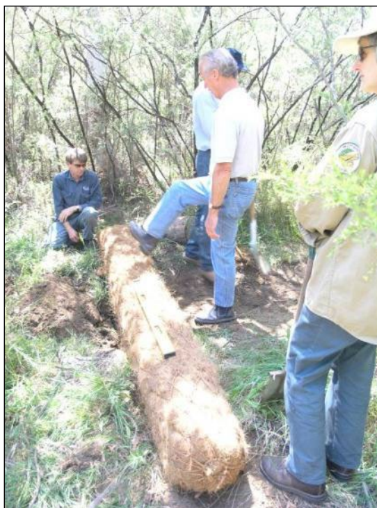
Figure 6-6 Round coir logs installed to spread water
