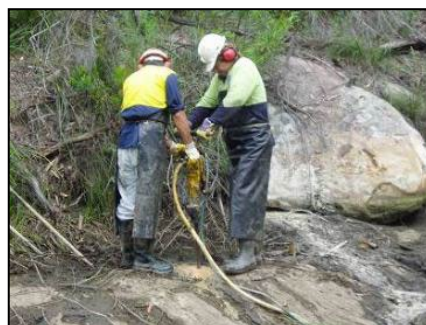
(b) Grout pump station setup
