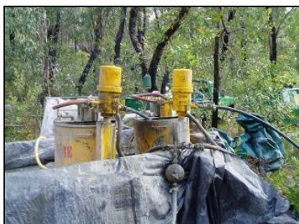
(a) Drilling into the bedrock
