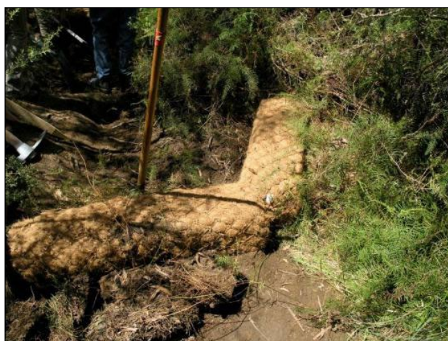
Figure 6-2 Square coir logs for knick point control
