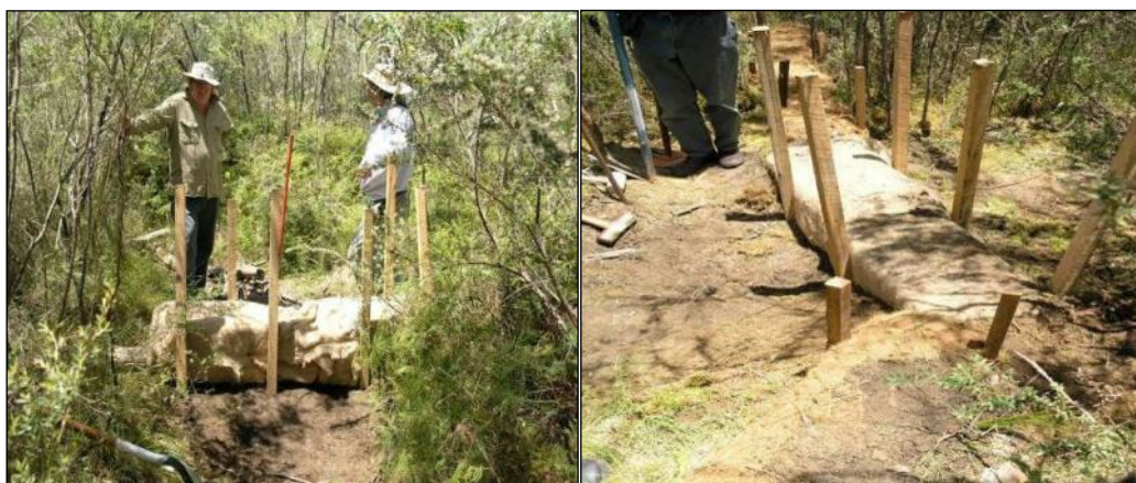
Figure 6-3 Installation of square coir logs
