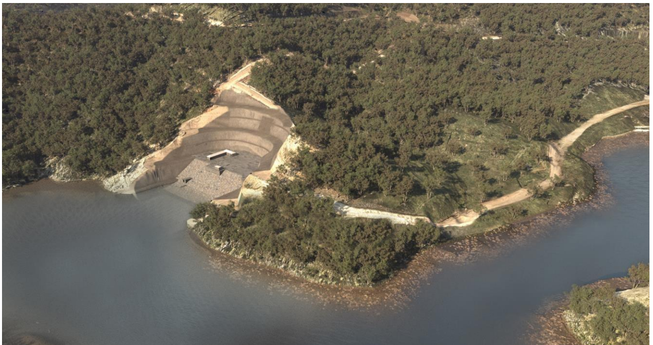
Figure C-1: Talbingo Intake Structure
