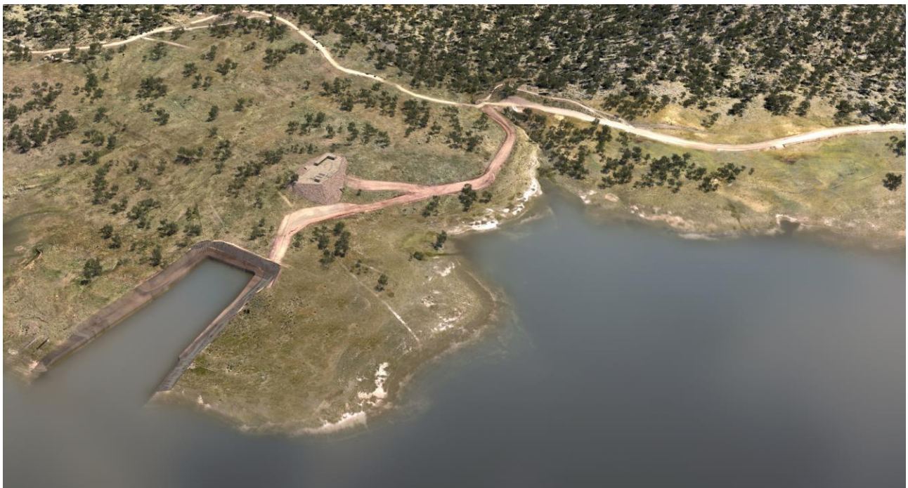
Figure D-1: Tantangara Intake Structure
