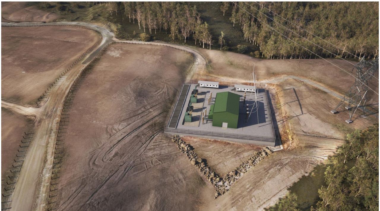
Figure A-1: Lobs Hole Substation – after construction
