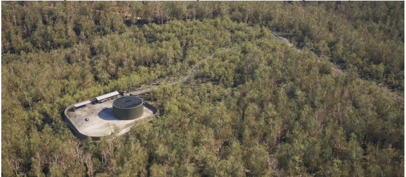
Figure E-1: Headrace Surge Shaft (aerial view from the east)
