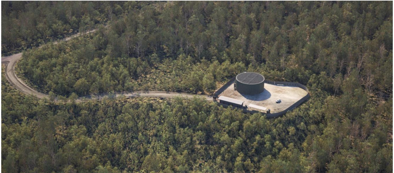
Figure E-2: Headrace Surge Shaft (aerial view from west)
