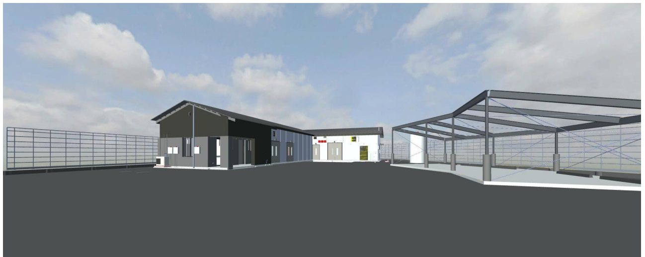
Figure D-3: Tantangara Intake Building north-east
