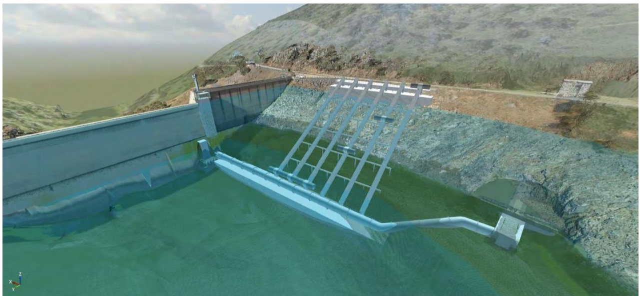
Figure F-1: Tantangara Fish screen concept design
