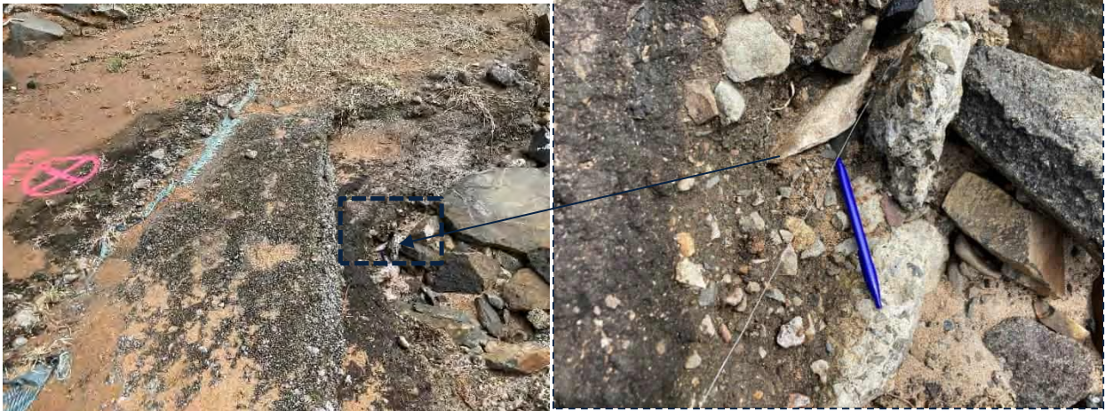
Photo 2-19 Example of ACM fragment observed protruding from eroded embankment wall near BH08 (Chainage 80m)
