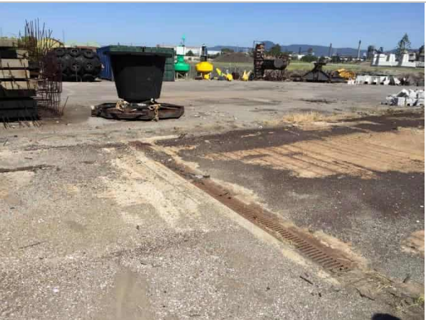
Photo 2-5 Looking west showing strip drains at edge of concrete slab (March 2021)
