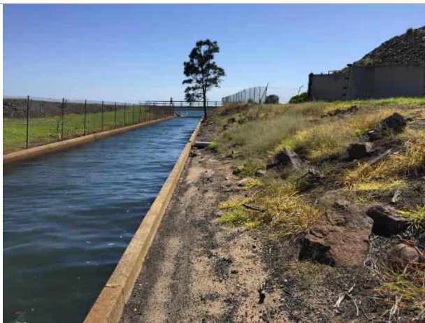
Photo 2-3 Looking north along the stormwater channel (March 2021)
