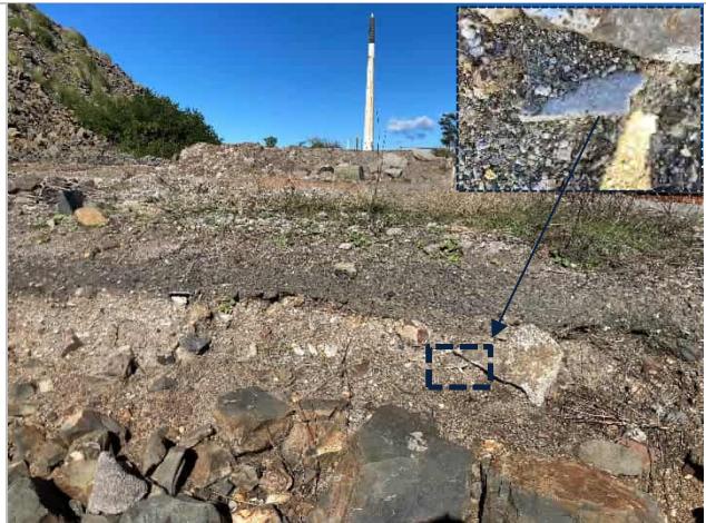
Photo 2-10 Evidence of ACM observed along eroded bank near stormwater outlet (April 2022)
