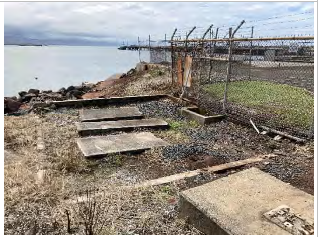
Photo 2-16 Concrete bunded area offsite north of BH06 (Chainage 180m)
