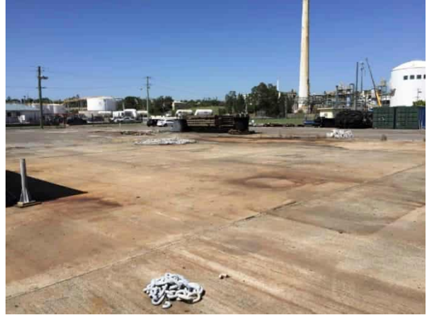
Photo 2-2 Looking south west along concrete slab area (March 2021)
