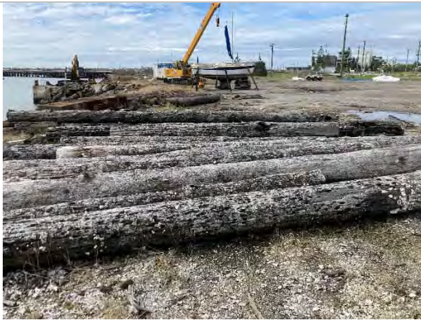
Photo 2-20 Timber poles stockpiled near BH07 (Chainage 110m)
