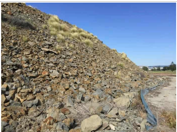
Photo 2-4 Looking west at surface of stockpile (March 2021)
