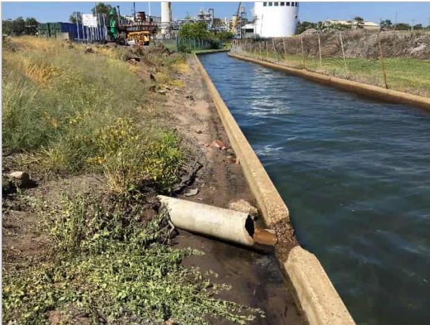
Photo 2-9 Buried ACM pipe observed on channel bank (March 2021)
