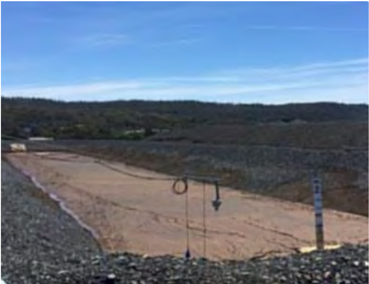
Figure D-1 Example of sludge lagoon at Clarence Colliery
