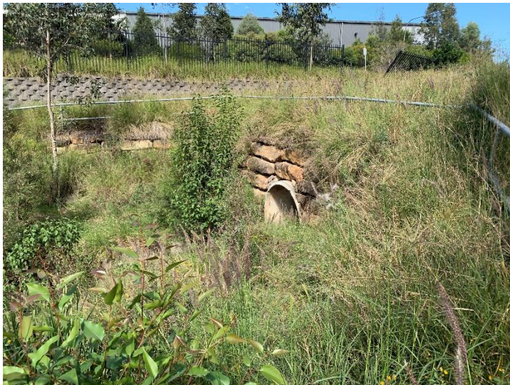
Photograph 6 Angus Creek at the Kangaroo Avenue culvert
