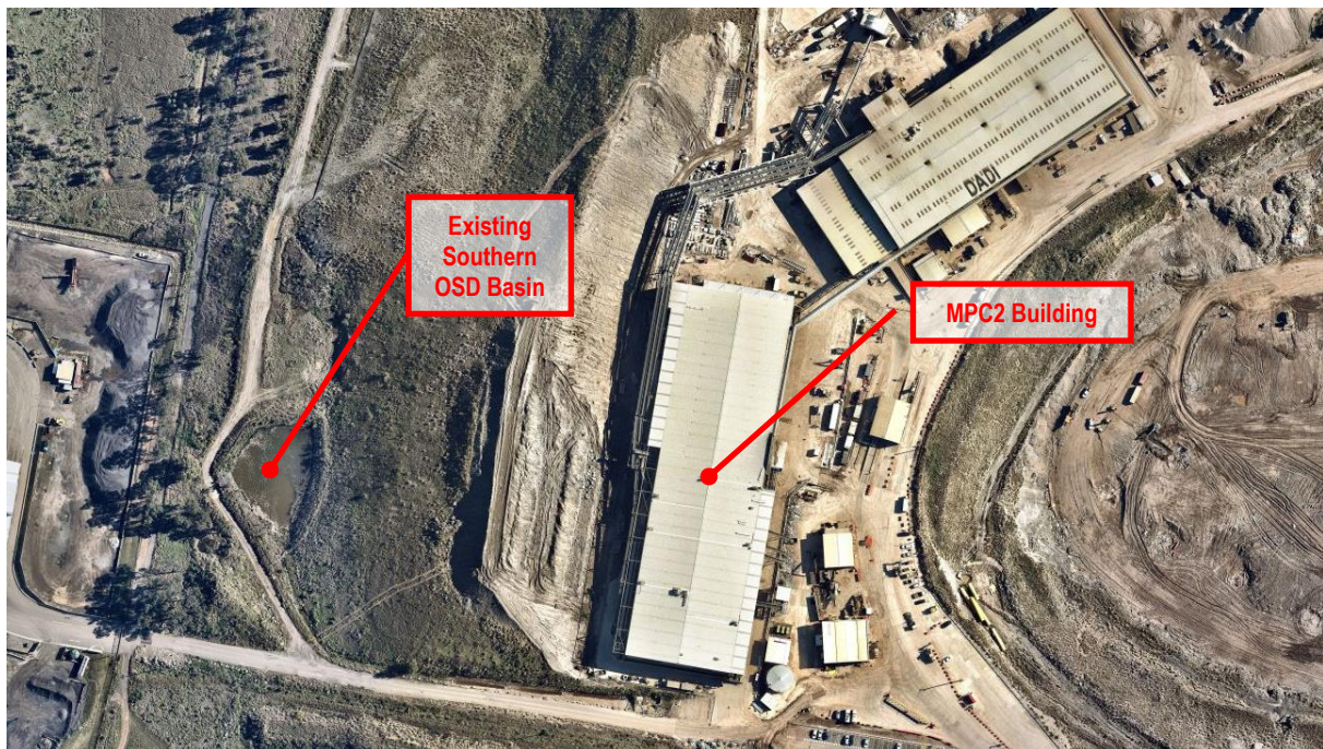
Figure 13: Existing Southern OSD Basin (nearmap, 17 October 2021)
