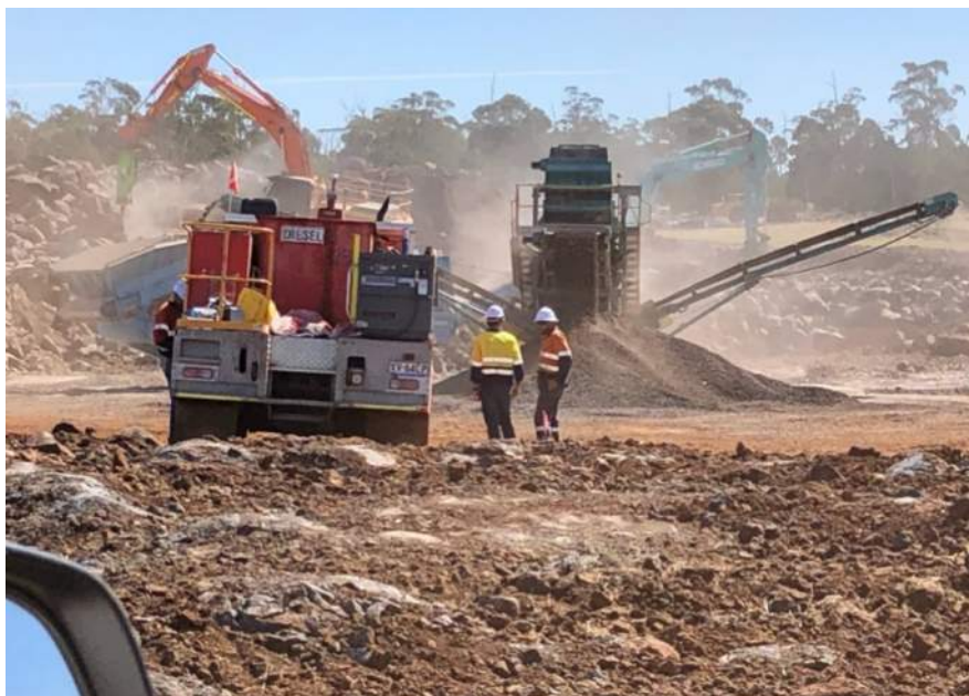
Figure 6: Crushing Circuit within On-Site Quarry.
