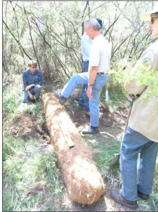
Figure 6-6 Round Coir Logs Installed to Spread Water
