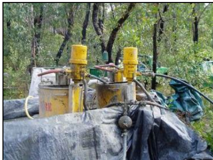
(a) Drilling into the bedrock
