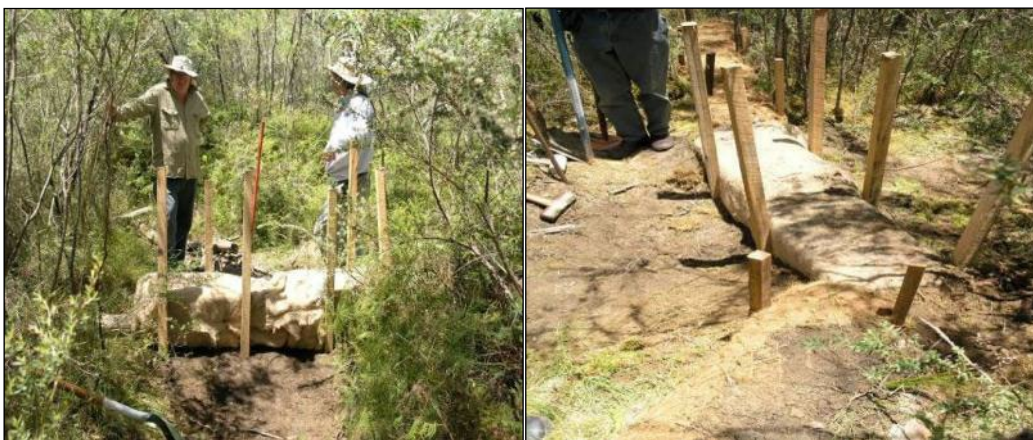
Figure 6-3 Installation of Square Coir Logs
