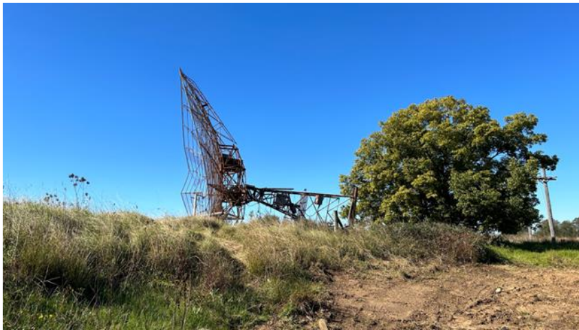
Figure 48 Antennae remnants full view on site
