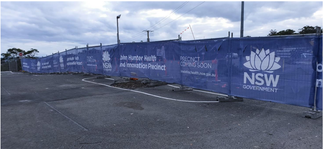
Photograph 10 – Fence wrapping JHH carpark
