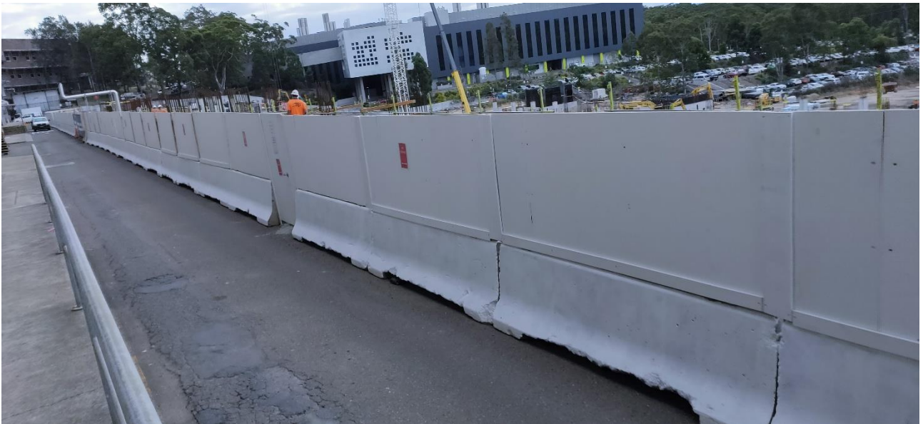
Photograph 9 – Hoarding on Kookaburra Circuit
