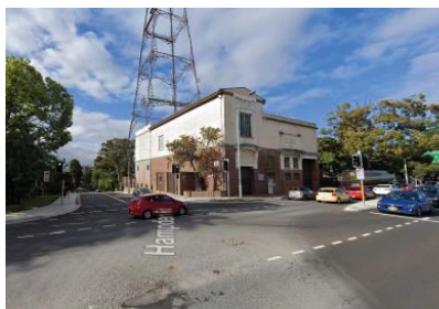
② Electricity Substation - Heritage listed
