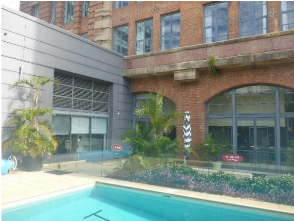
Figure 3 – The contemporary addition and interface with the former vehicle dock opening
