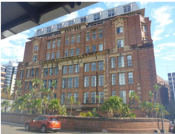
Figure 1 – East elevation as viewed from the YHA Railway Square. Note the brick retaining wall that defines the rear yard.
