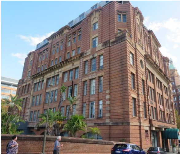
Figure 7 – View to east elevation from within the railway square.
