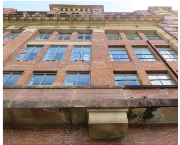
Figure 8 – View directly to the eastern elevation from within rear yard.
