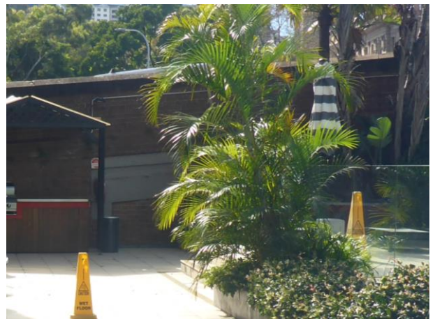
Figure 6 – View north showing the yard wall and evidence of the infill of the former access and level changes
