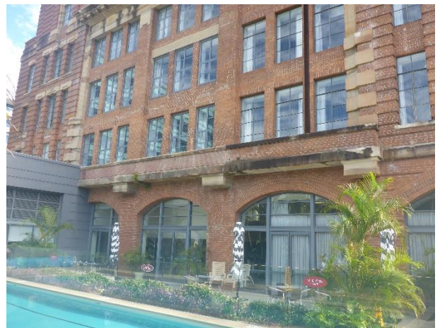
Figure 2 – The former vehicle dock openings on the east elevation have been infilled with aluminium framed glazing/ doors
