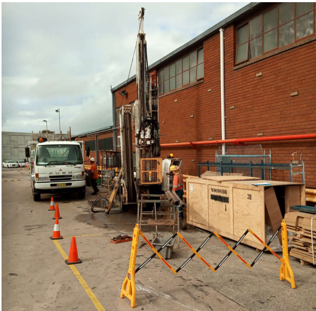
Photo 5 - Drilling rig and exclusion zone
