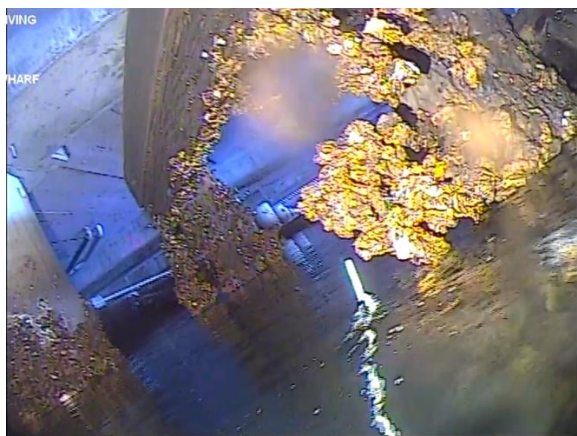
Figure 58: Timber stormwater baffle; 'D' pile to the left of image. Note large hole in net and missing timbers from baffle. (Image from T2 (a) Cockle Bay 210705, 03:57).
