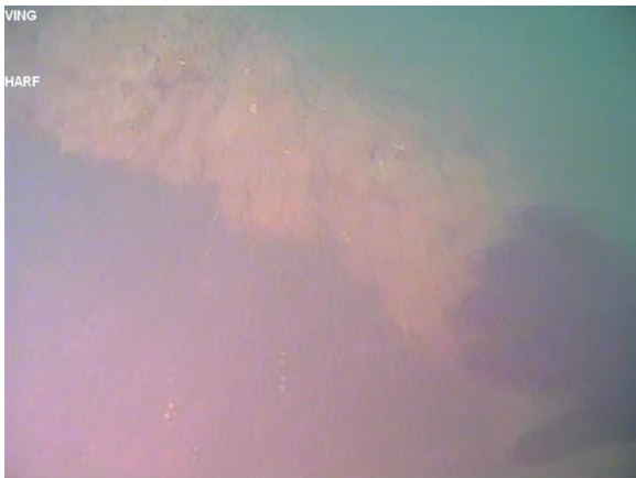
Figure 94: Rectangular pile on a 45° angle to the south in the centre of the bent adjacent to 'A' pile at the western end of T8. (Image from T8 (d) Cockle Bay 210705; 08:07).
