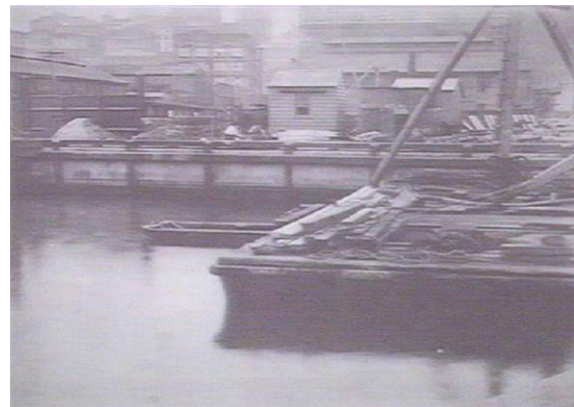
Figure 42 : Completed Monier plate facing of seawall between Wharves 35 and 36, Darling Harbour, 1919. 45
