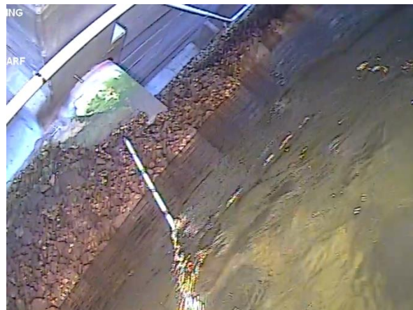
Figure 85: Southern 'D' pile is out of the water behind the sheet piling wall. (Image from T6 (a) Cockle Bay 210705).
