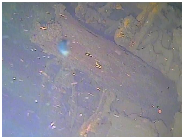
Figure 97: Timber pile adjacent to 'B' pile in centre of bent and surrounded by construction debris. (Image from T9 (a) Cockle Bay 210705; 03:06).
