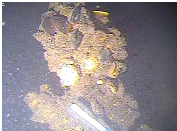
Figure 104: Heavily deteriorated cut off timber pile 1500 mm to the south of the northern 'E' pile. (Image from T10 (b) Cockle Bay 210705; 05:00).
