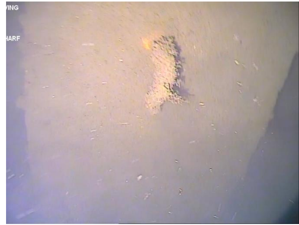
Figure 52: Modern concrete mooring block between steel piles 'B' and 'C' on the southern side of T1. (Image from T1 (a) Cockle Bay 210705; 03:38).
