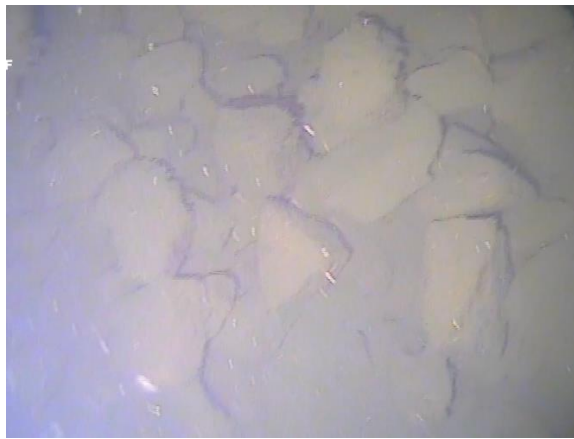
Figure 86: Rock batter emerging from the sediment to the east of the 'B' pile. (Image from T7 (b) Cockle Bay 210705; 01:12).
