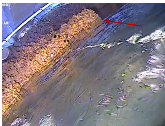
Figure 74: Sheet pile wall 1.5 m behind 'D' pile. The sheet pile returns to the east to run into the sea wall at the red arrow. (Image from T4 (a) Cockle Bay 210705, 07:06).
