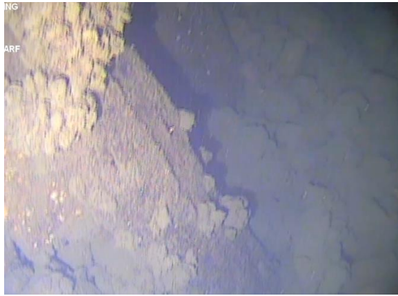
Figure 100: Two of the cut off timber piles near the southern 'E' steel pile. (Image from T10 (a) Cockle Bay 210705; 07:39).
