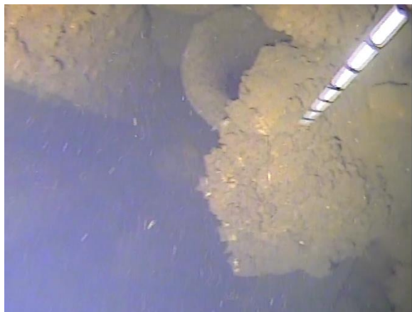
Figure 90: Degraded and hollowed out timber pile northeast end of transect 7. (Image from T7 (b) Cockle Bay 210705; 03:56).
