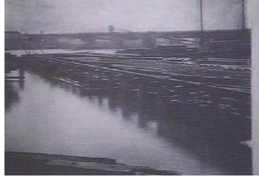
Figure 21: Wharf 35 under construction, September 1918. 28
