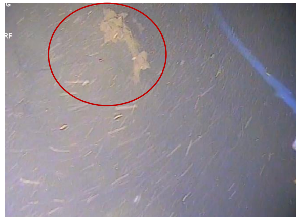
Figure 103: Top of the northern cut off timber pile closest to the northern 'E' steel pile. Note heavy deterioration. (Image from T10 (b) Cockle Bay 210705; 02:52).
