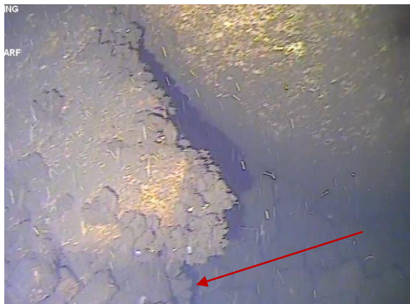
Figure 102: Rectangular piece of concrete leaning against southern 'E' pile. Timber pile underneath indicated by red arrow. (Image from T10 (a) Cockle Bay 210705; 09:01).
