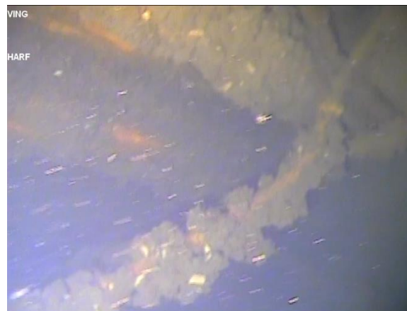
Figure 69: Sheet piling in background with loose ferrous piping in the foreground. (Image from T3 (a) Cockle Bay 210705, 07:38).
