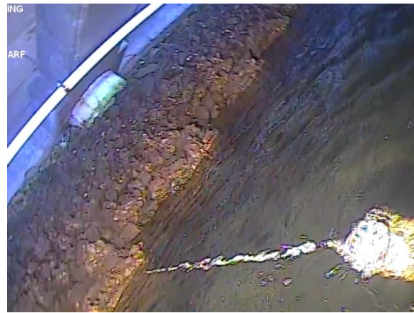
Figure 87: Sheet pile wall at eastern end of transect holding up rock batter. (Image from T7 (b) Cockle Bay 210705; 02:17).
