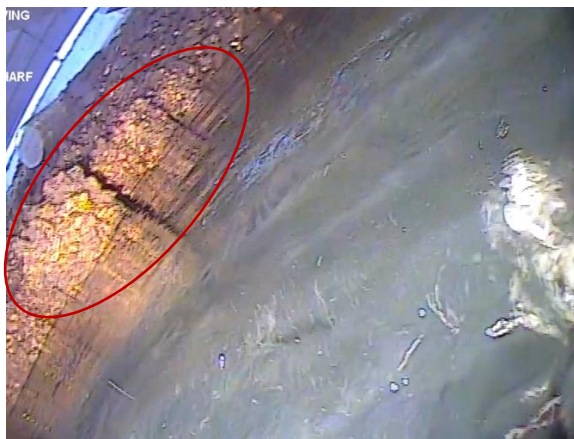
Figure 68: Sheet piling appears to start in this bent. (Image from T3 (a) Cockle Bay 210705, 07:49).
