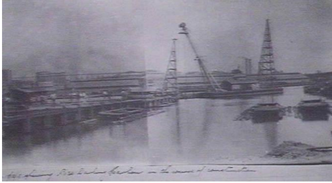
Figure 20: Wharf 36 under construction, December 1918. 27
