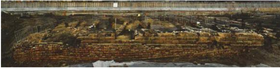
Figure 7: Sandstone seawall at Barangaroo South, identified through archaeological excavation by Casey and Lowe 48
