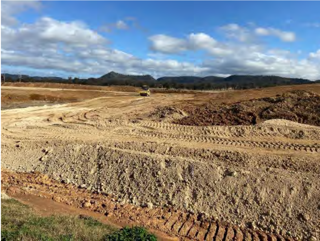
Plate 21 – MCCO Sed dam 2 embankment construction 22 July 2022
