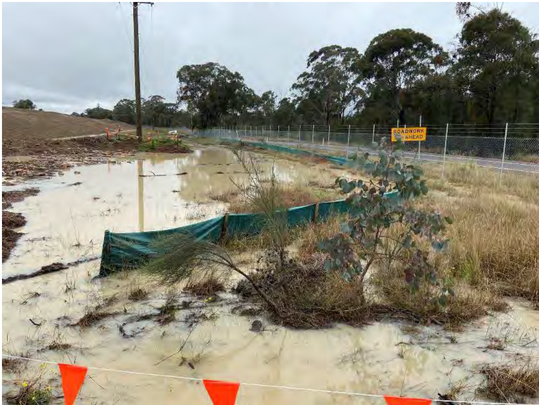
Plate 11 – MCCO sediment controls in place during site inspection on 5 July 2022.
