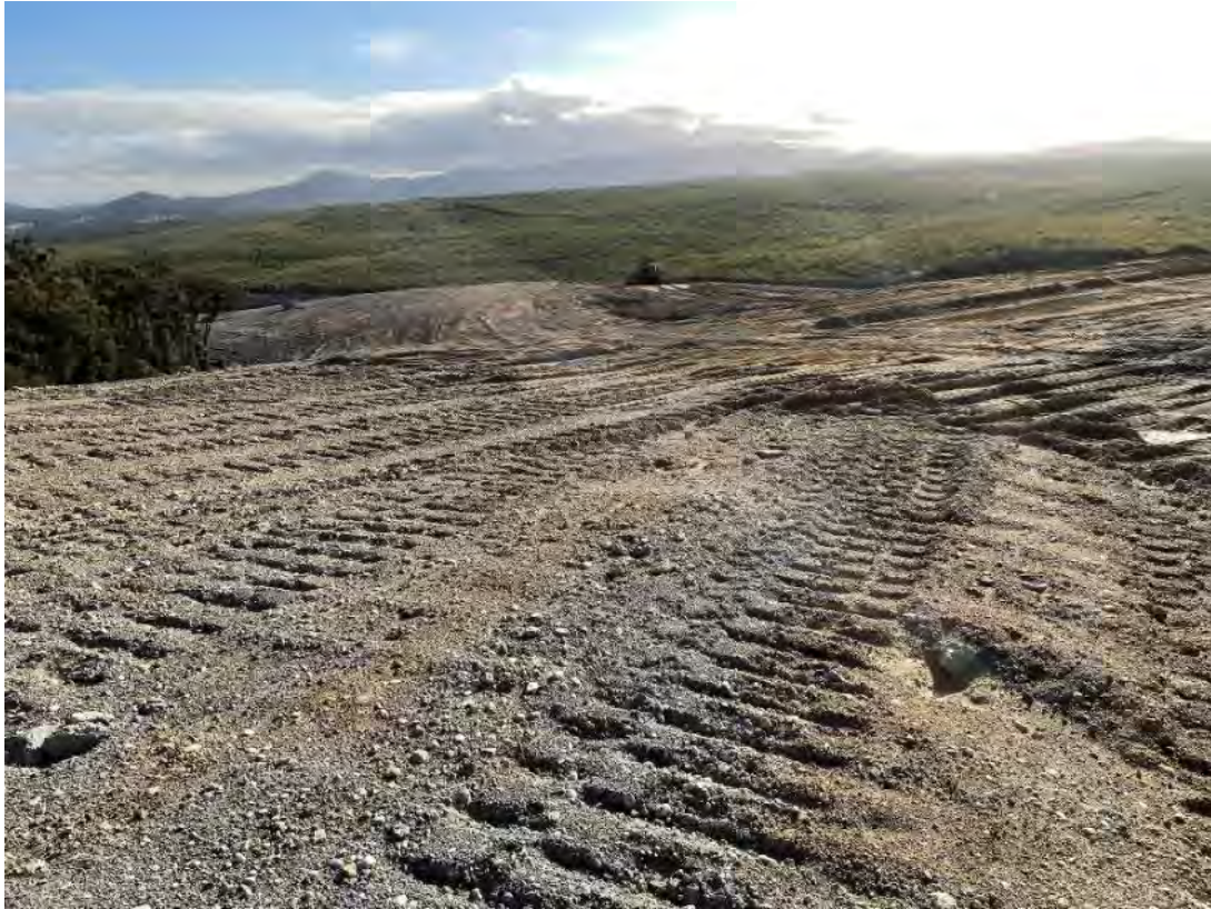
Plate 31 – Low profile geomorphic landform being constructed.
