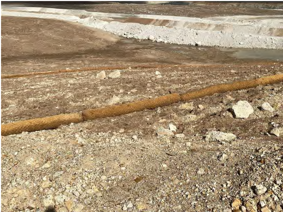
Plate 37 – Temporary erosion control to minimise rilling on temporary rehabilitation area.
