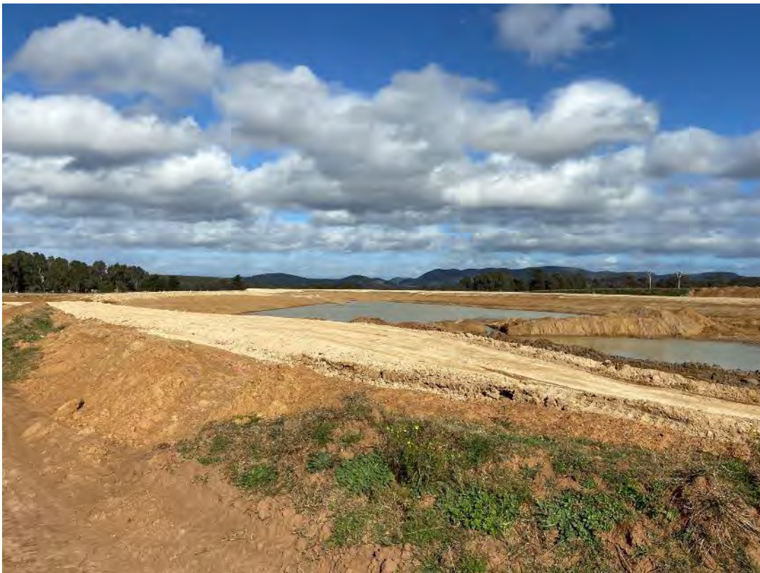
Plate 22 – MCCO Sed dam 2 construction 22 July 2022
