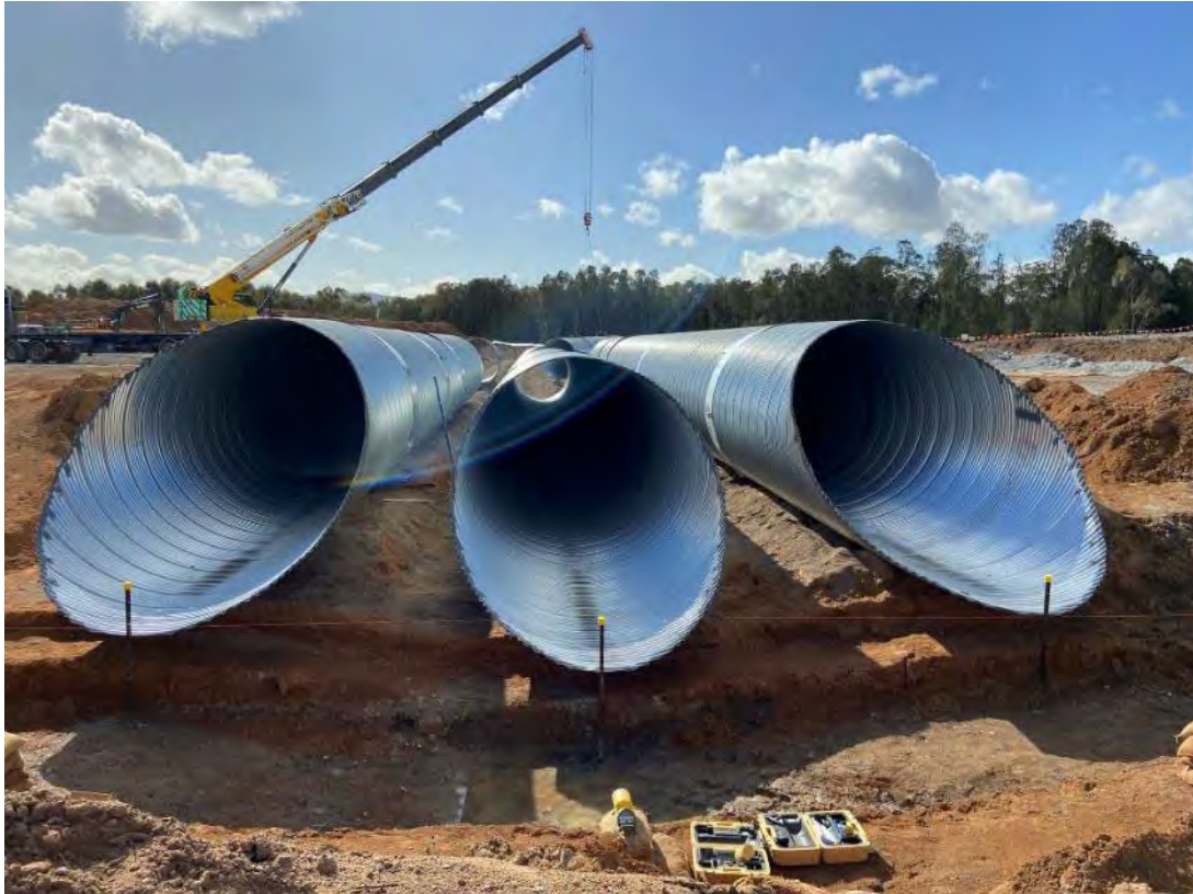
Plate 29 – Big flat creek permanent (life of project) drainage diversions pipes
