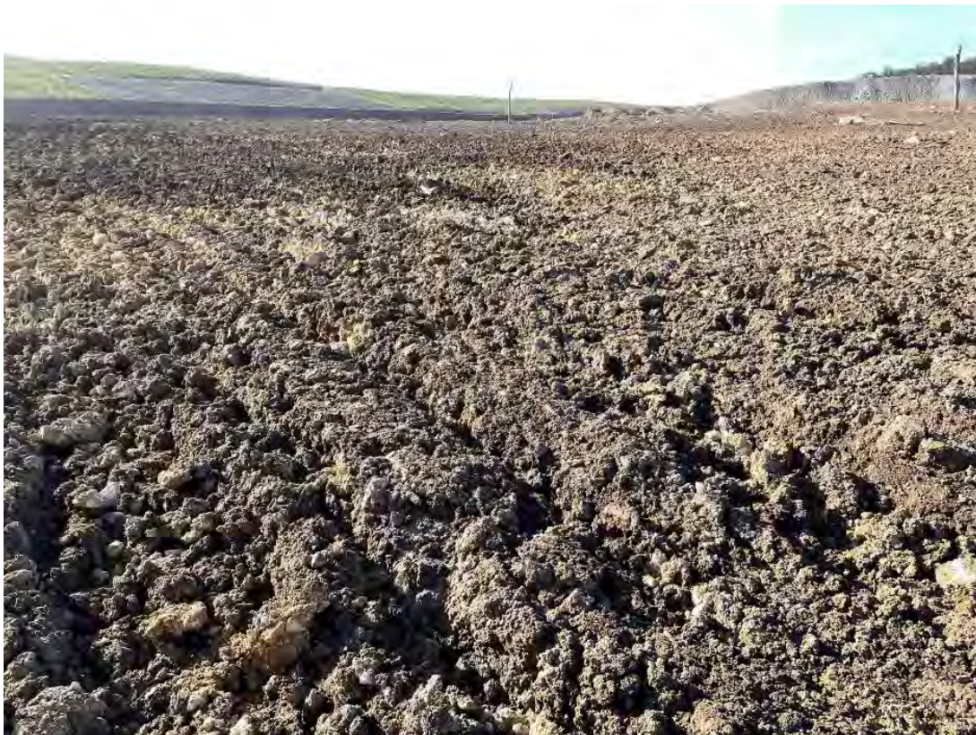
Plate 32 – Deep ripping on contour surface prep prior to seeding.
