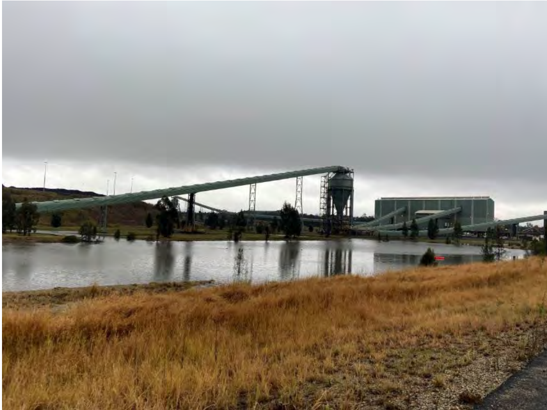
Plate 5 – CHPP and anvil creek storage dam during site inspection 5 July
