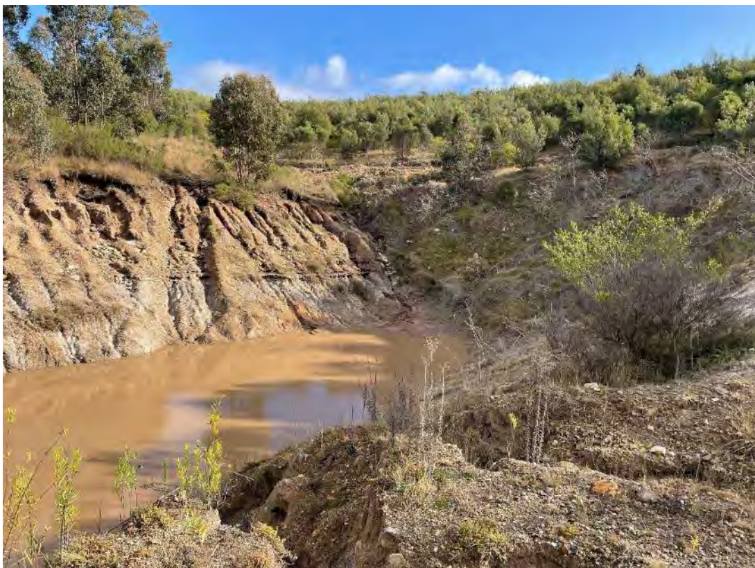
Plate 24 – South Pit South Sediment Dam with eroding banks creating turbid water. Runoff from the upslope catchment has been monitored and is of a good quality. Hence recommendation is to rehabilitate dams to allow for potential offsite release of water to reduce the mine water generation during wet periods (currently pumped back into the mine water system).
