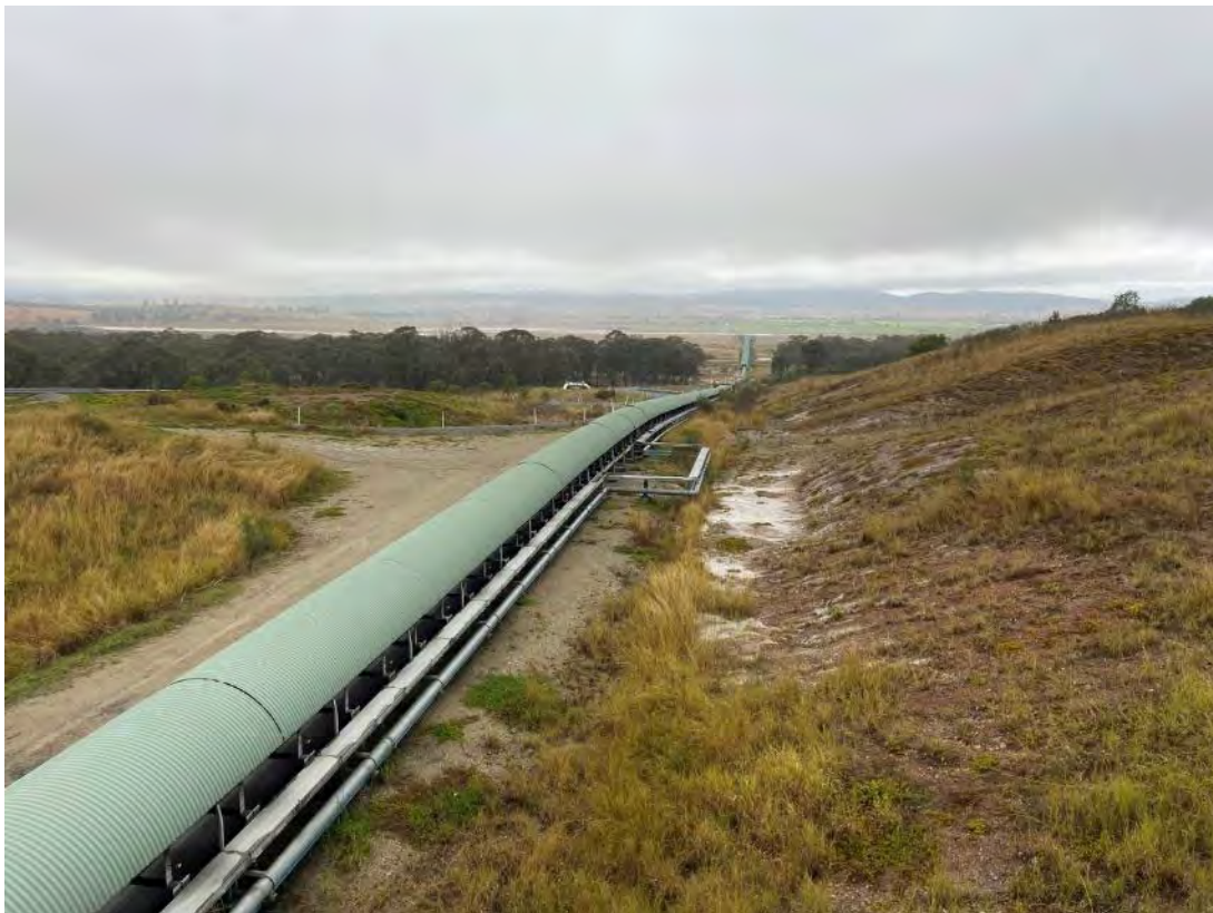
Plate 4 – Covered conveyor belts observed on site during site inspection 5 July
