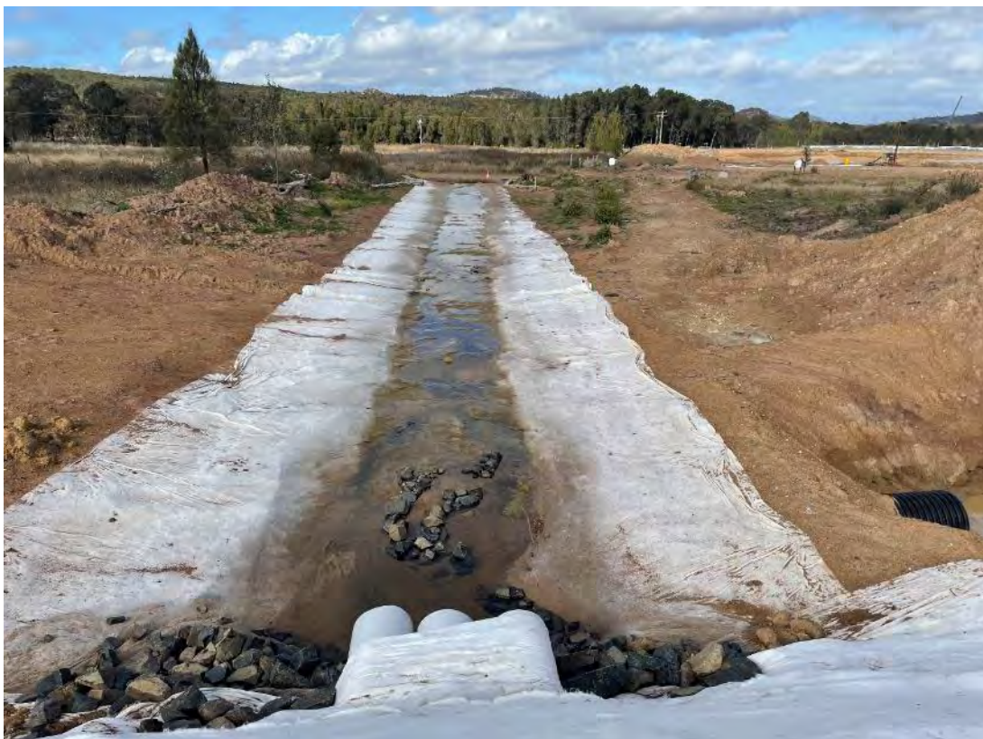
Plate 26 – Temporary clean water diversion in place for the MCCO project
