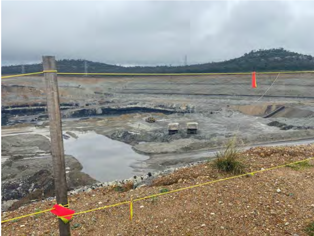
Plate 1 – Active mining area during site inspection 5 July 2022.
