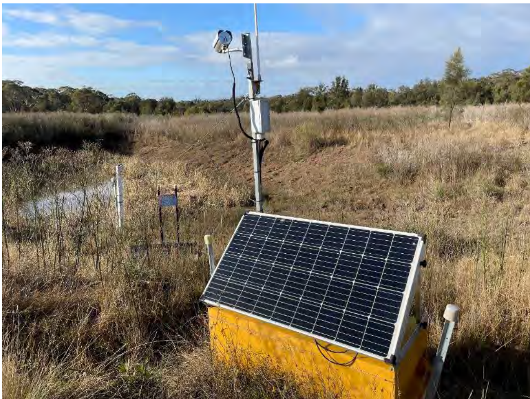
Plate 28 – Sand Creek Farm Dam Automatic Level Sensor Monitoring Equipment
