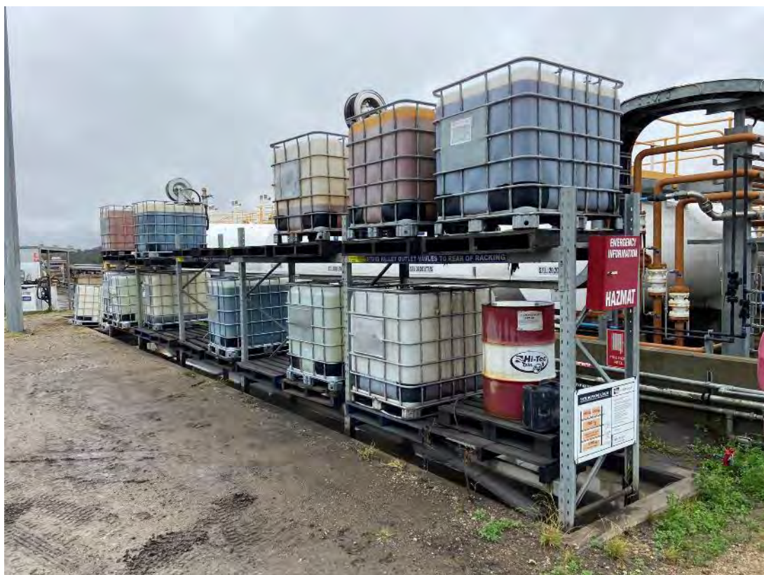
Plate 18 – Chemical storage on adequately bunded areas.
