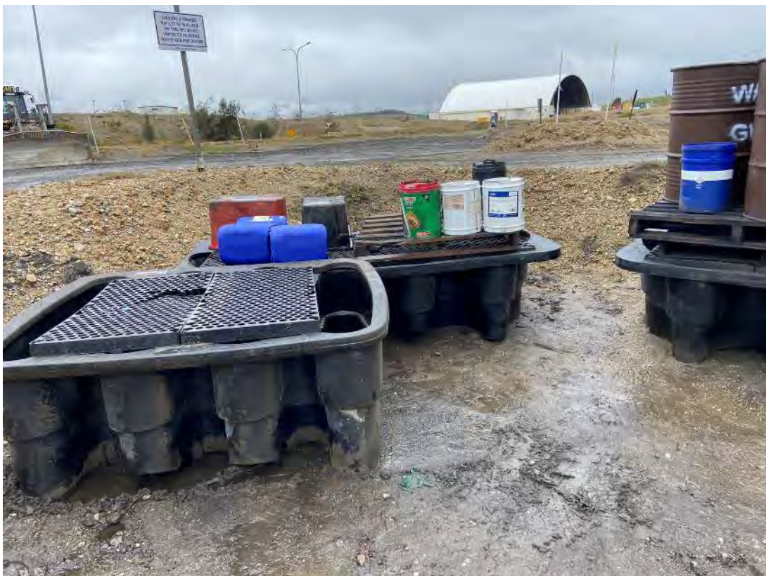
Plate 16 – Waste chemicals stored on bunded structures
