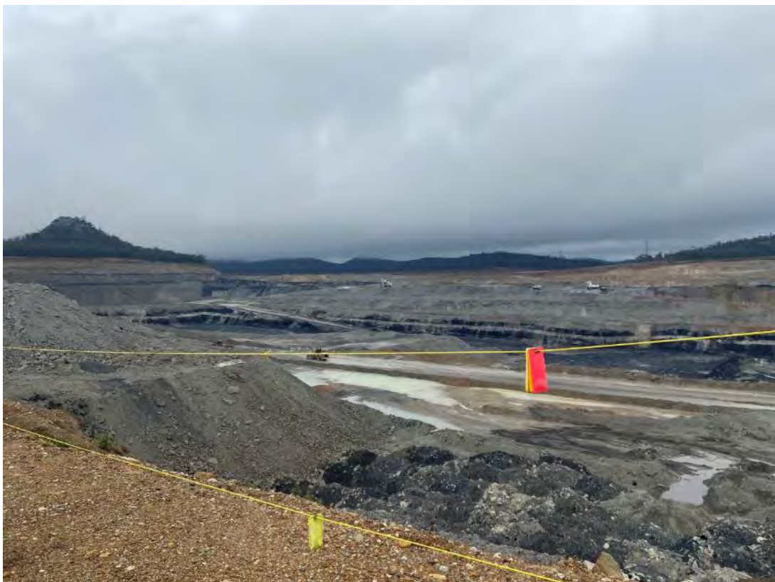
Plate 2 – Active mining area during site inspection 5 July 2022, Anvil Rock (left).
