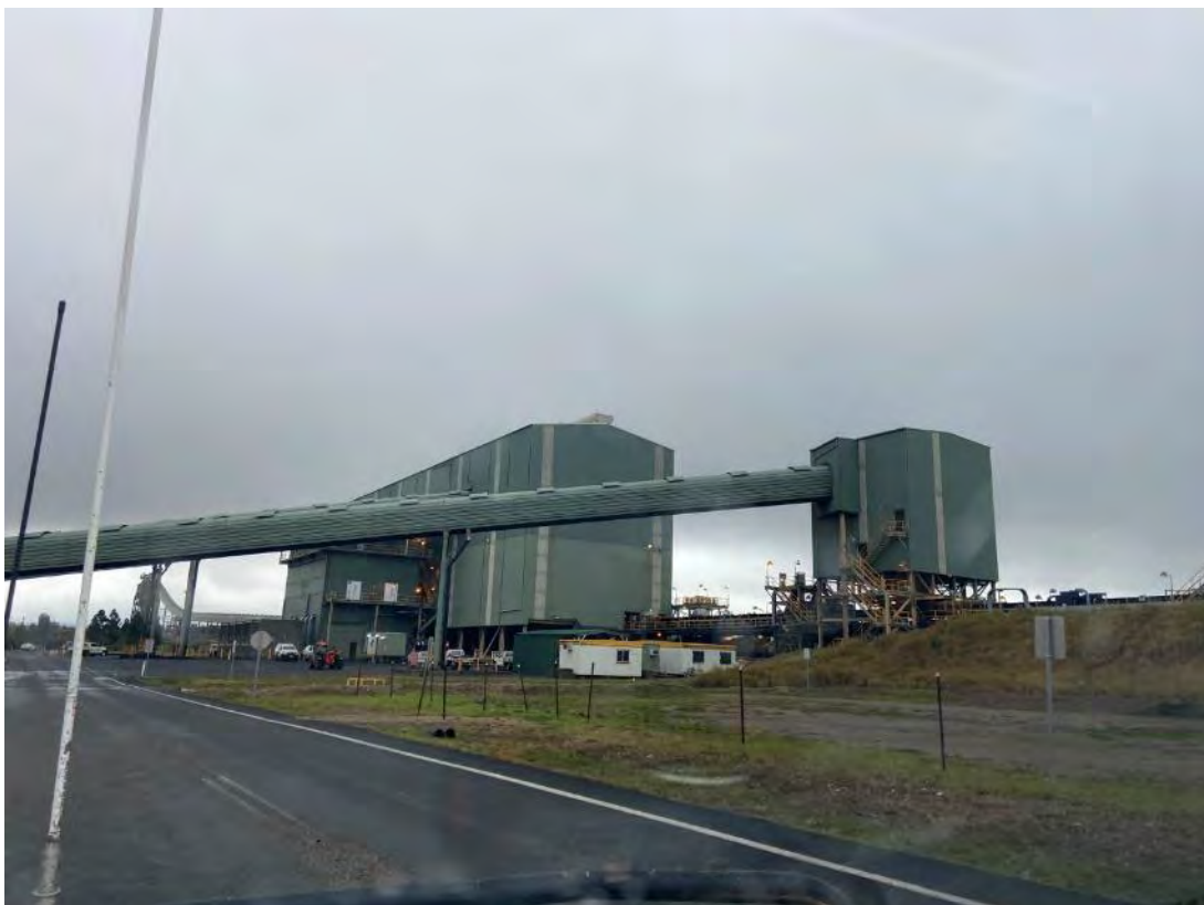
Plate 6 – CHPP during site inspection 5 July
