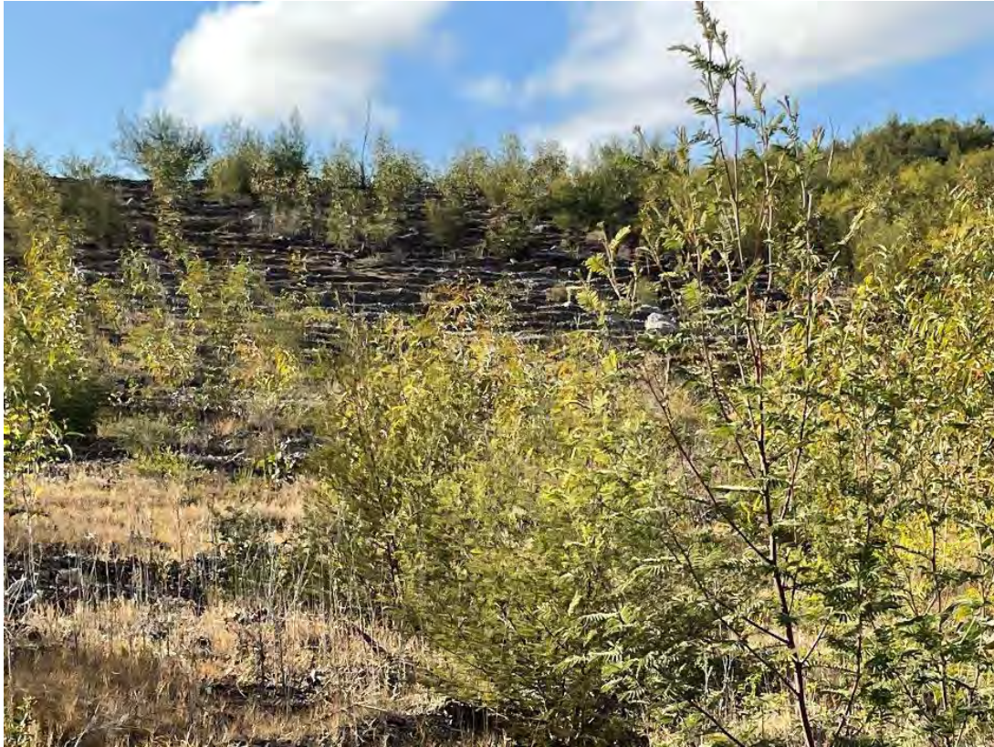
Plate 33 – Old Erosion gully repaired, ripped and seeded.
