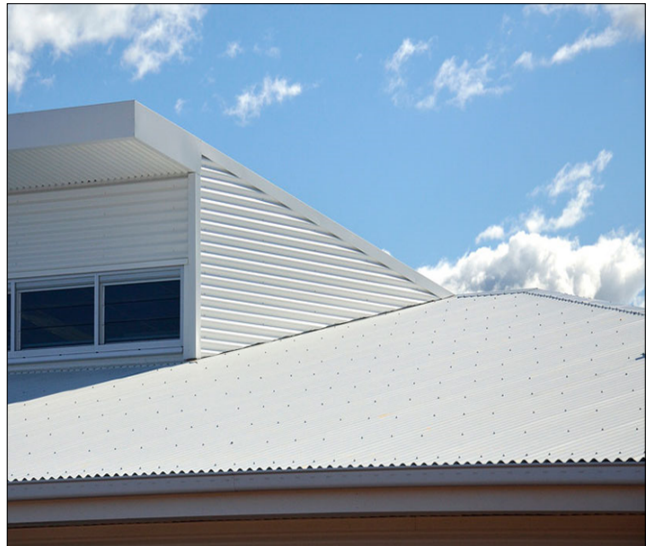
Figure 9 - Illustration of a light coloured (reflective) roof sheeting.
