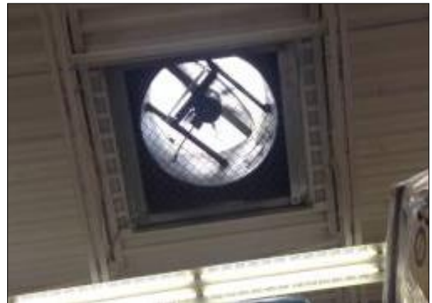
Figure 12 - Motorised smoke exhaust fans can enable hot air to escape through roof, facilitating air ventilation.
