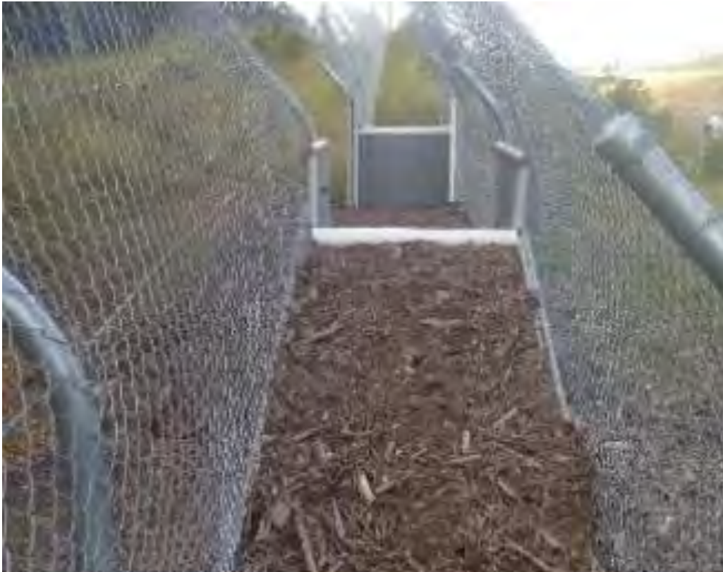
Plate 6 Escape ramp with 1.2m drop to not allow Koala access into the fence but can safely drop out to safe area.
