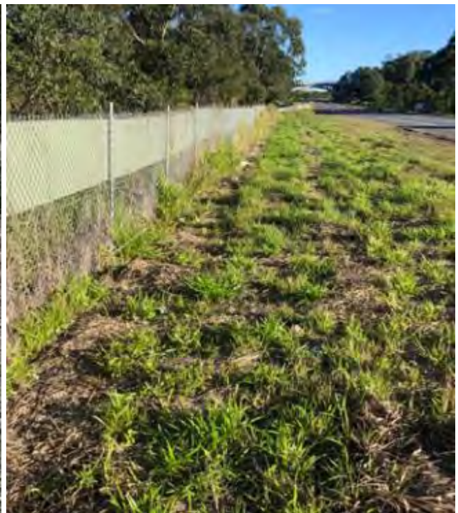
Plate 5 1.5m Fencing with 600mm metal flashing
