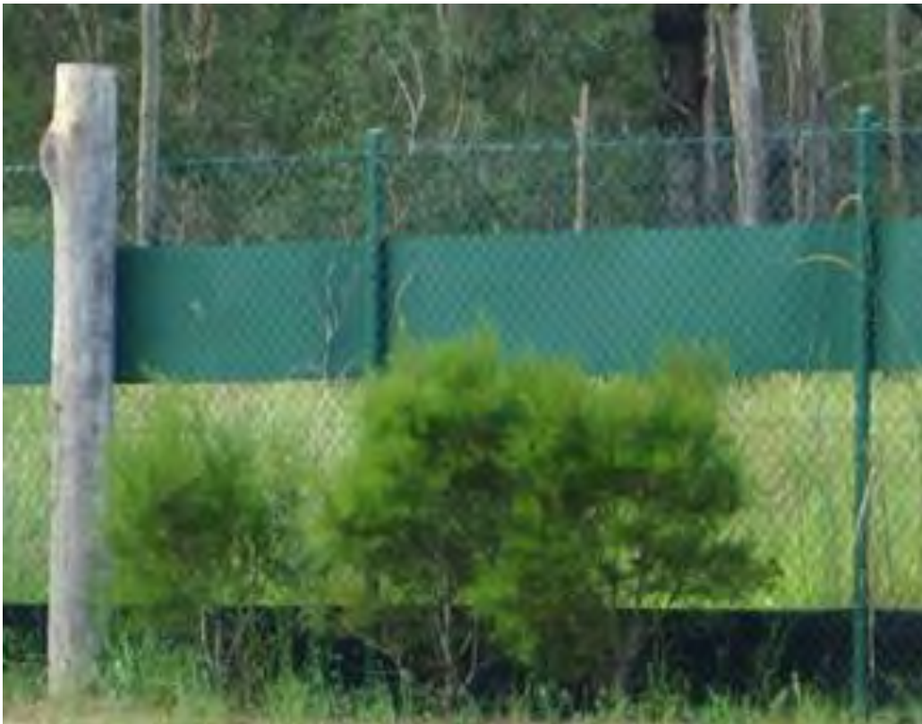
Plate 7 Escape pole for Koala from inside the fence into safe areas.
