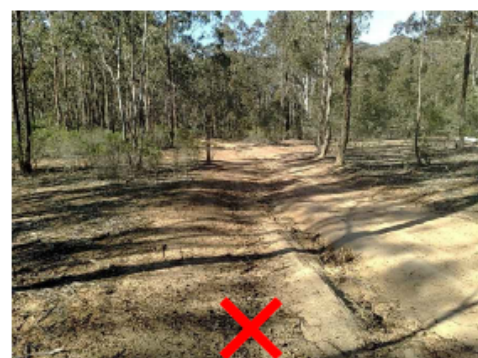
WHEEL RUTS FUNNEL WATER ALONG TRACK, CAUSING EROSION
