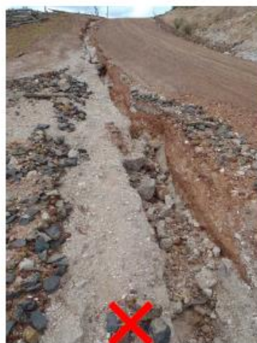
LACK OF STABLE DRAINAGE ON A STEEP SECTION OF TRACK
