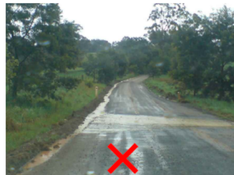
UNCONTROLLED DRAINAGE. WATER SPILLS ACROSS TRACK AT LOW POINTS, CAUSING EROSION
