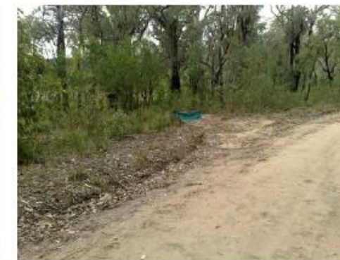
SEDIMENT FENCES SHOULD NOT BE REQUIRED IN TURN-OUT DRAINS IF THEY ARE CONSTRUCTED PROPERLY
