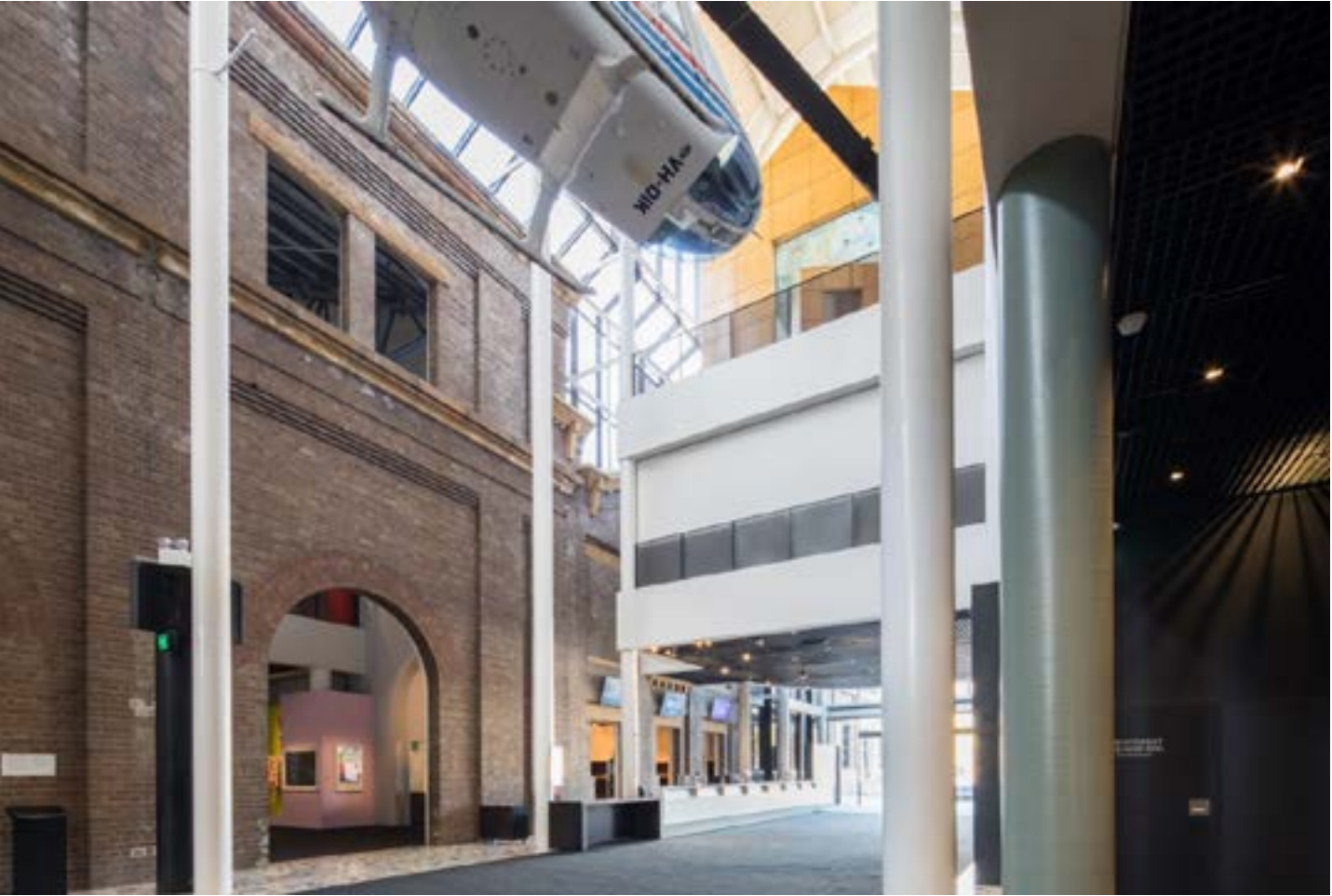
Figure 11.15 Turbine Hall western façade, now integrated as an internal wall within the Museum (Source: Powerhouse)
