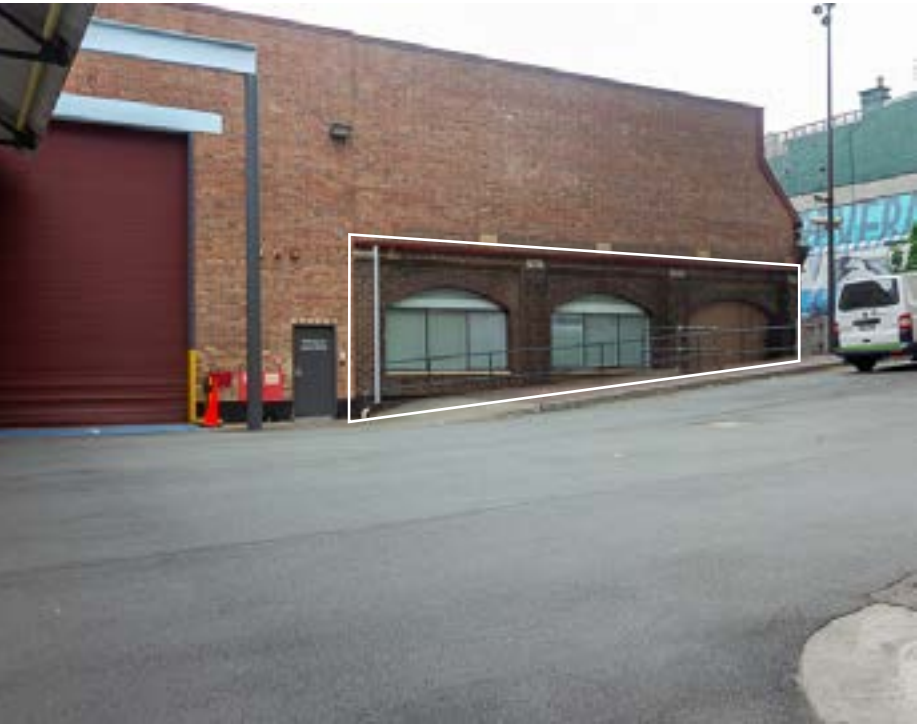
Figure 7.28 The northern wall of the Harwood building, original brickwork around windows in white (Source: Curio Projects)
