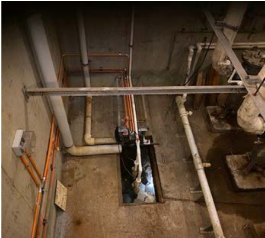
Figure 16.10 Sea water return pit (Source: Powerhouse)
