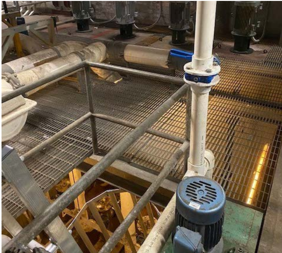
Figure 16.9 Sea Water pump pit suction motors (Source: Powerhouse)
