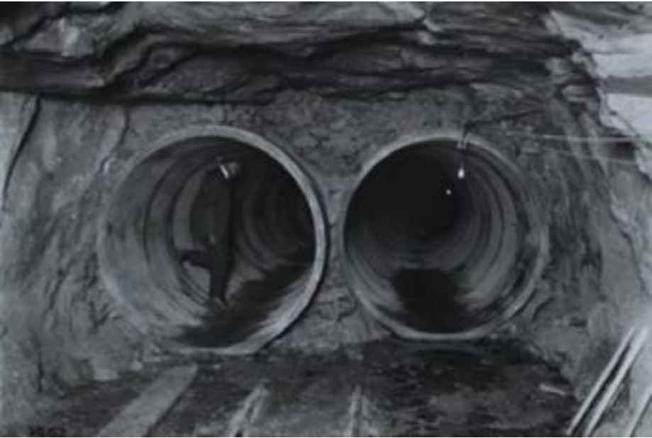
Figure 16.4 Close up of Water conduits with man for scale. Rails in the foreground were used to cart rubble to fill the space between the two pipes. (Source: State Rail NSW Item 364/46)
