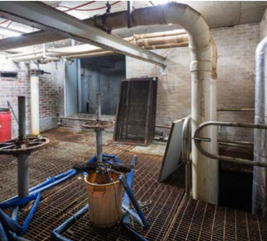
Figure 16.8 Sea Water pit and penstock valve (Source: Powerhouse)
