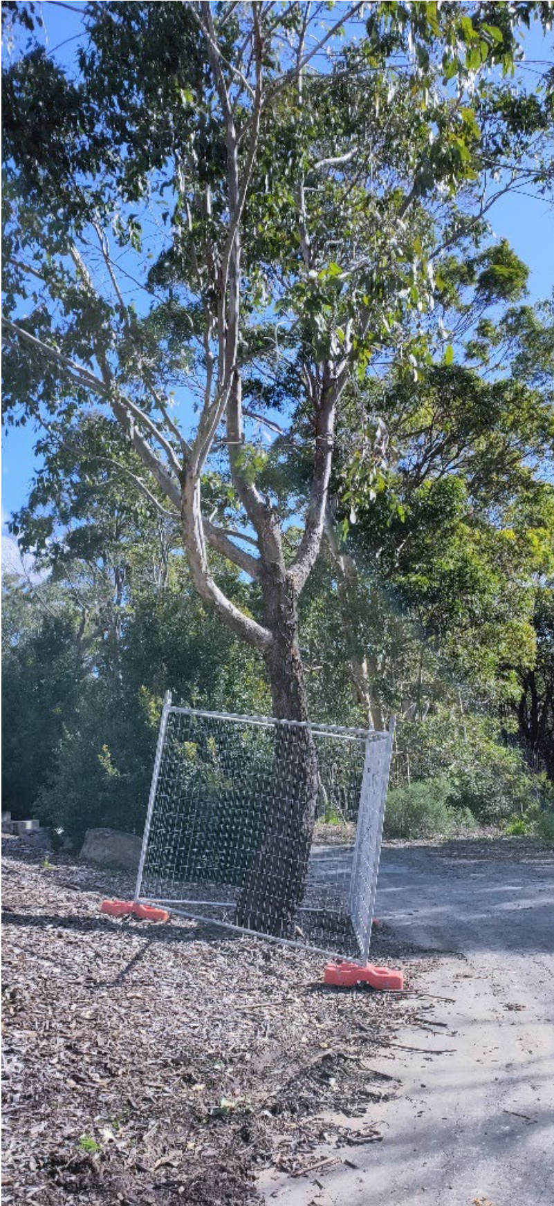
Photograph 13 – Tree protection around retained tree
