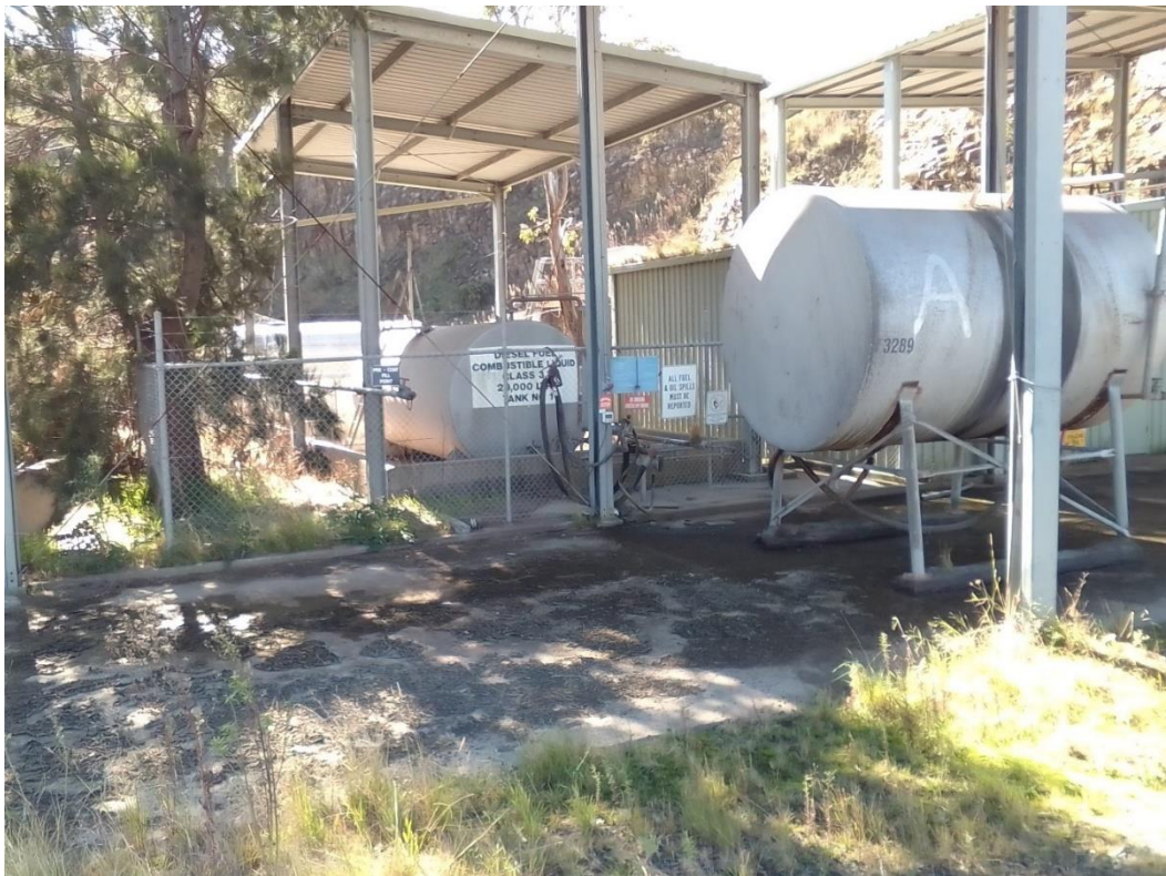
Plate 1 Hydrocarbon Storage Tanks and Storage Area within the quarry site
