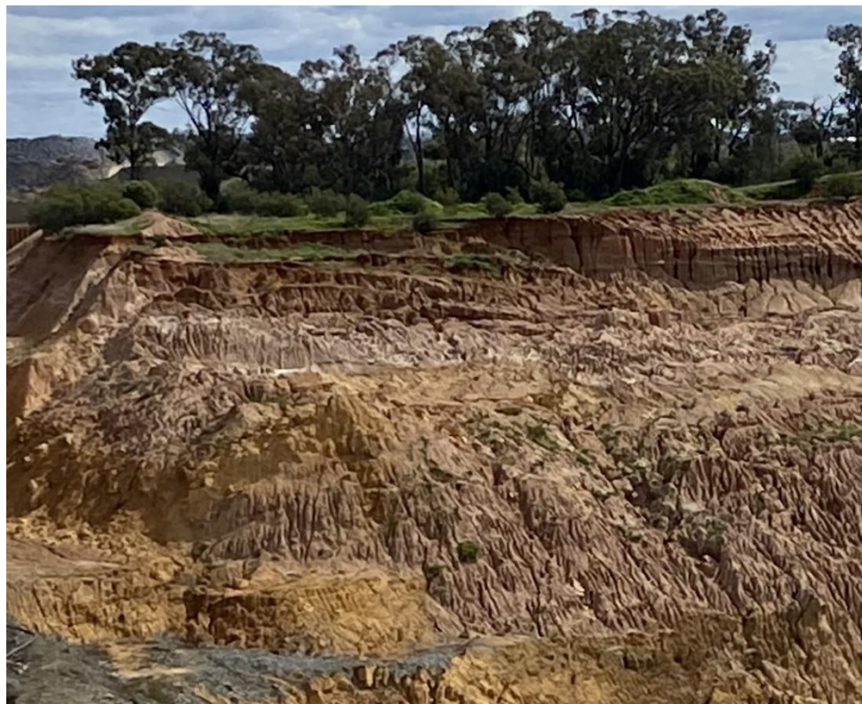
Figure 4: Example of a regressive, multiple-slice slope failure in the western wall of the Caloma 1 pit.
