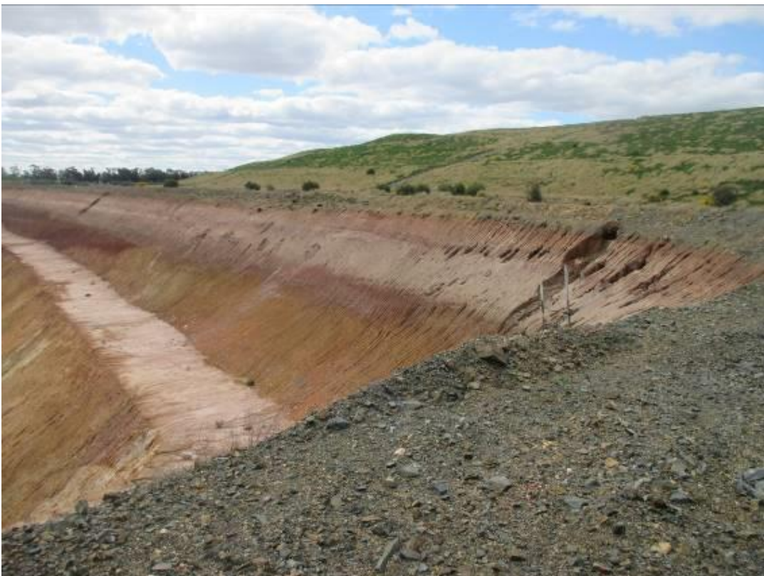
Figure 6: Caloma 1 Open Cut looking north-west (top) displaying structure and failures (top). Image displays a large gully with vertical sides and headcut. Bottom image (looking north) displays tunnel and gully erosion in the surface material. Of note is the tunnel through the bund.
