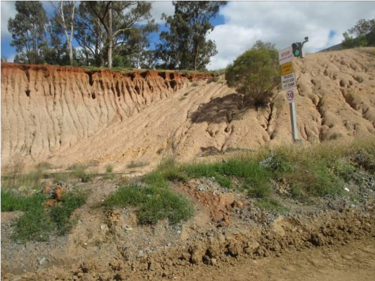
Figure 7: Cutting through natural material on southern side of mine road passing under the Newell Highway. Tunnel and rill erosion can be observed in the natural material on the left while large rills can be observed on the fill material (right) used as an abutment for the bridge.
