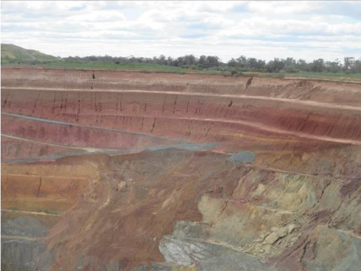
Figure 3: Wyoming 1 Open Cut looking north-west. A large mass failure (centre), and a smaller failure (right) can be observed. Tunnels from tunnel erosion and gullies can be observed in both alluvium and saprolite.
