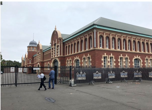
Figure 9 – View towards the south east corner of the building.
