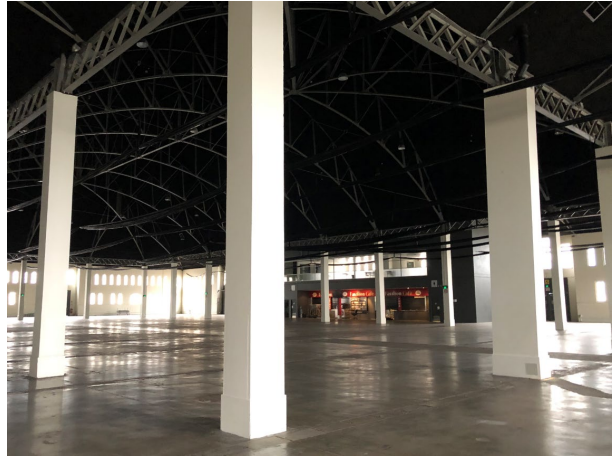
Figure 12 – View north east across internal space.
