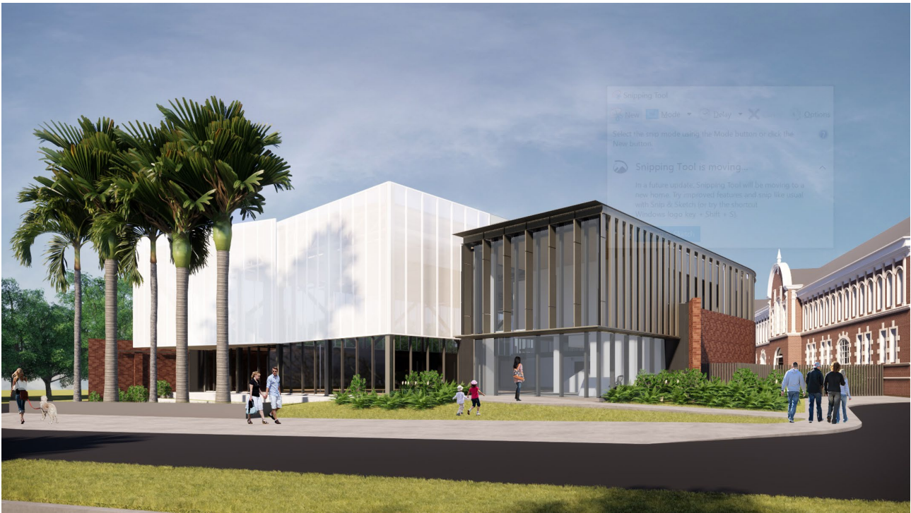
Figure 27 – NSW Swifts building
