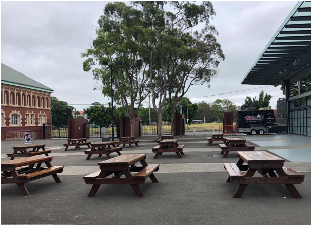
Figure 3 –Open space north of the building.
