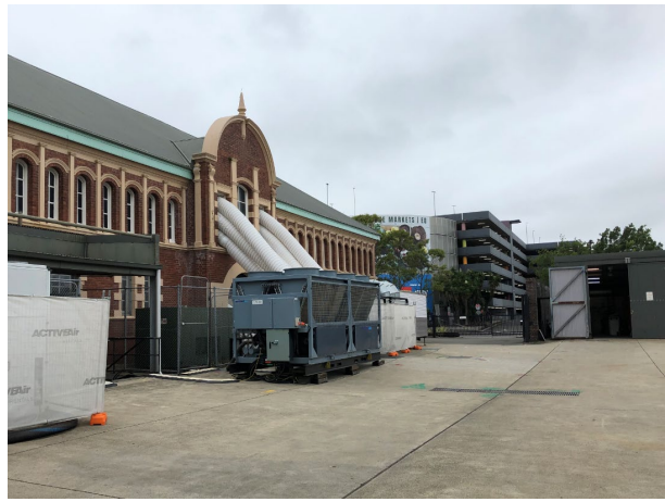
Figure 6 – View across open space to south of building showing temporary air conditioning measures.
