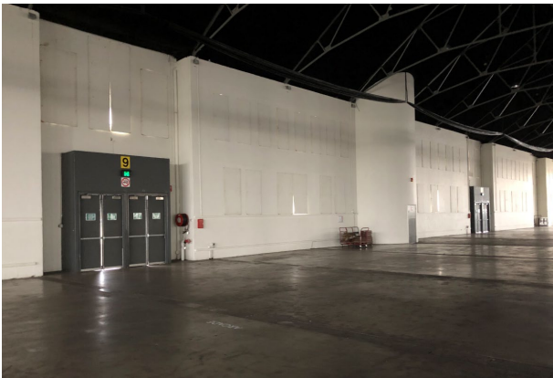
Figure 15 – View towards inside of door 9.
