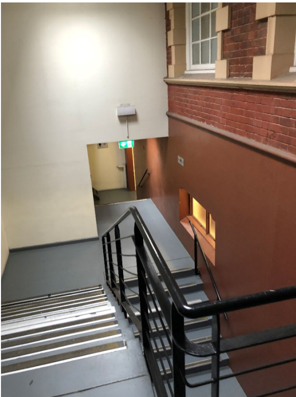
Figure 19 – View towards stair.
