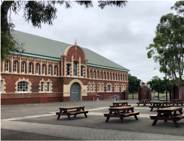
Figure 7 – Part view of north façade.
