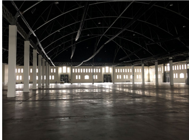
Figure 14 – View across internal space.
