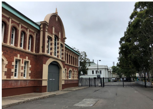
Figure 10 – Part view of east façade.
