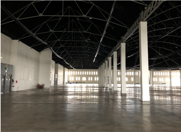
Figure 13 – View across internal space.
