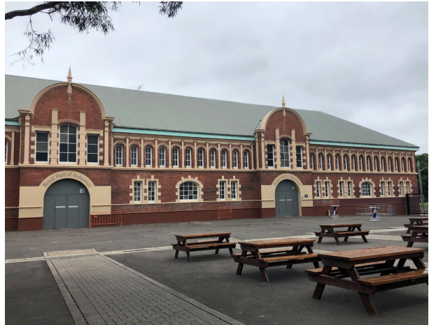
Figure 8 – Part view of north façade.
