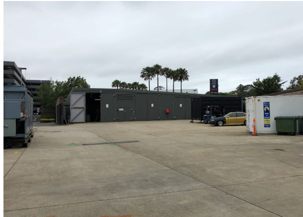
Figure 4 – View across open space to south of building.
