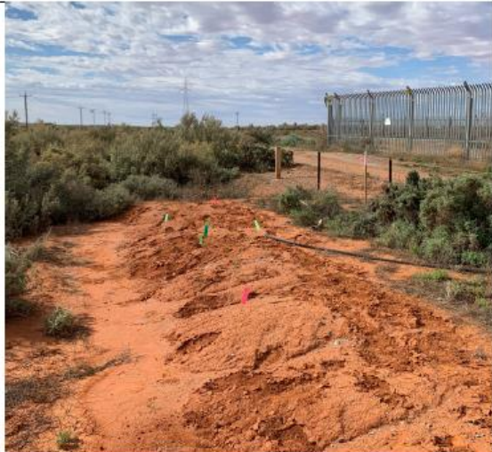
Plate 6 View southeast of BESS-AS1-21 (23-4-0691)
